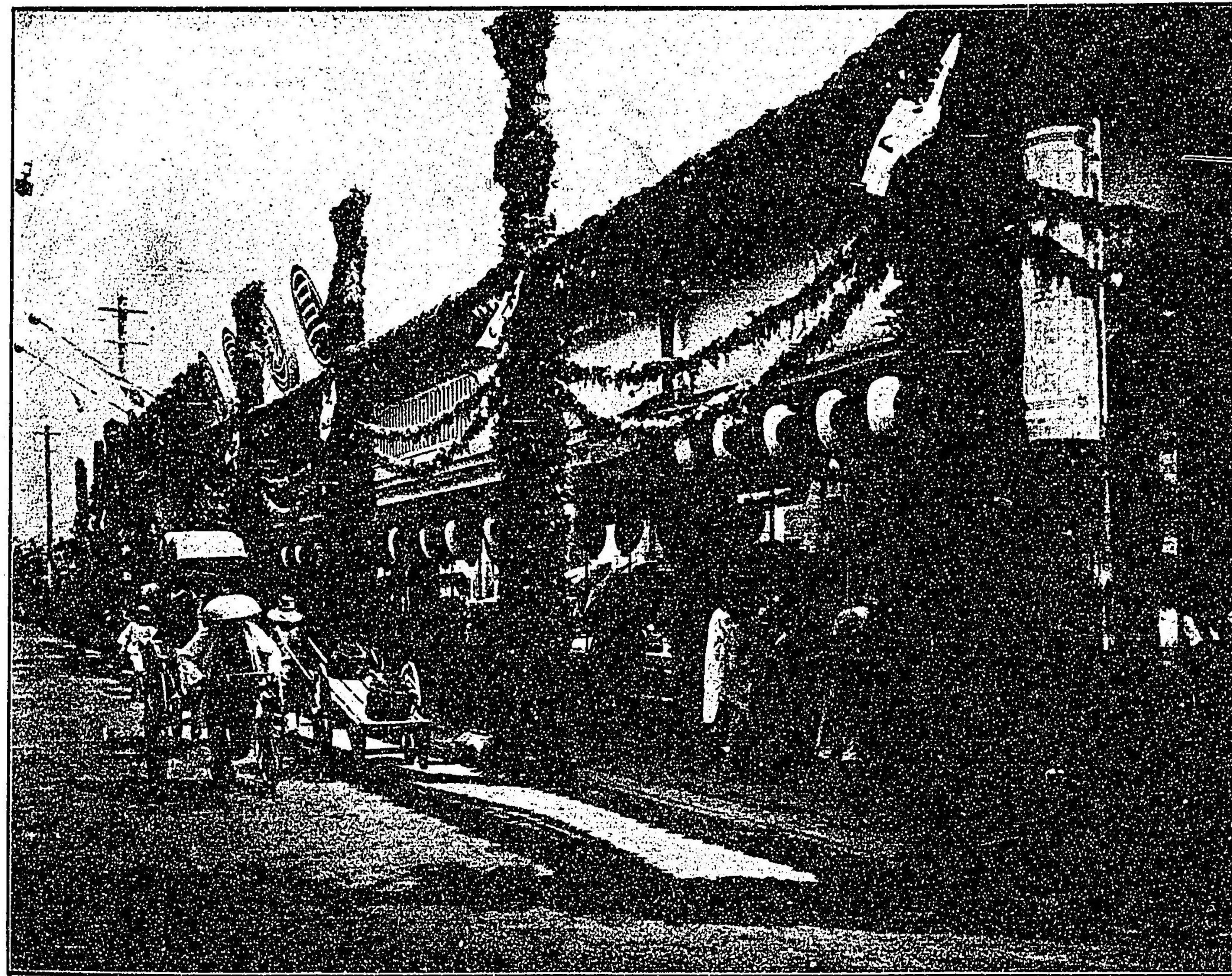
The Mitsukoshi Dry Goods Store,
