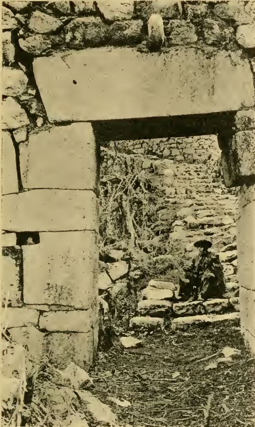
FIG. 5.—Machu Picchu. City gate, interior. Notice the lock hole containing granite cylinder on left and projecting ring stone over the lintel of the doorway. The gate, probably of wood, was either swung from the ring stone or fastened to it and balanced by a log fastened to the stone cylinders in the lock hole on either side of the gateway. A similar device was used also in the entrance doors to each isolated group of houses. Copyright by the National Geographic Society.
