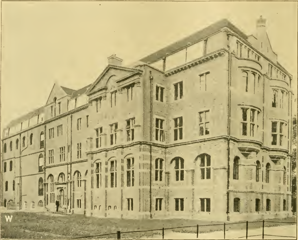
New Physiology School, Cambridge. View from N.W. The large lecture room and the biochemical department will form a wing on the E. side of the entrance door.
