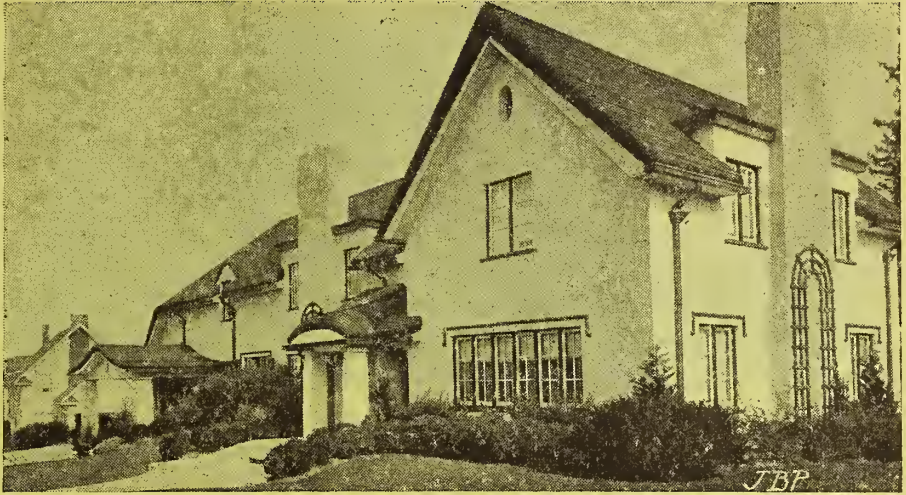
HOME WELL TIED TO GROUND
