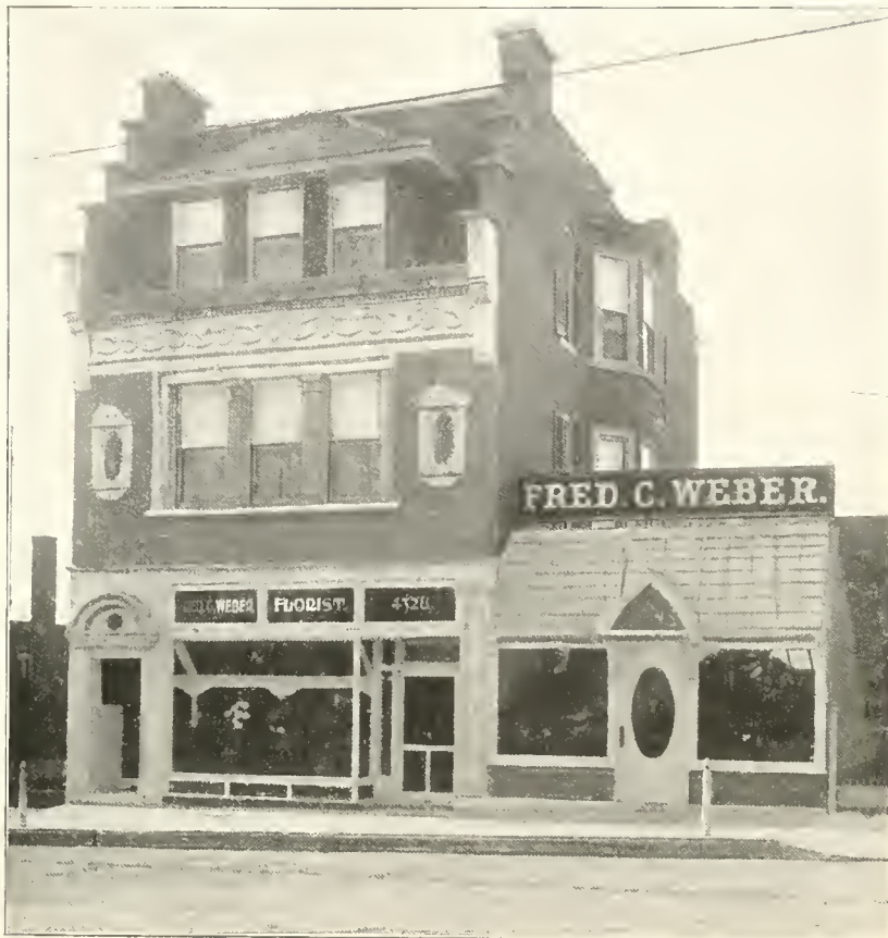
Exterior of the new store of Mr. Fred. C. Weber, St. Louis.
