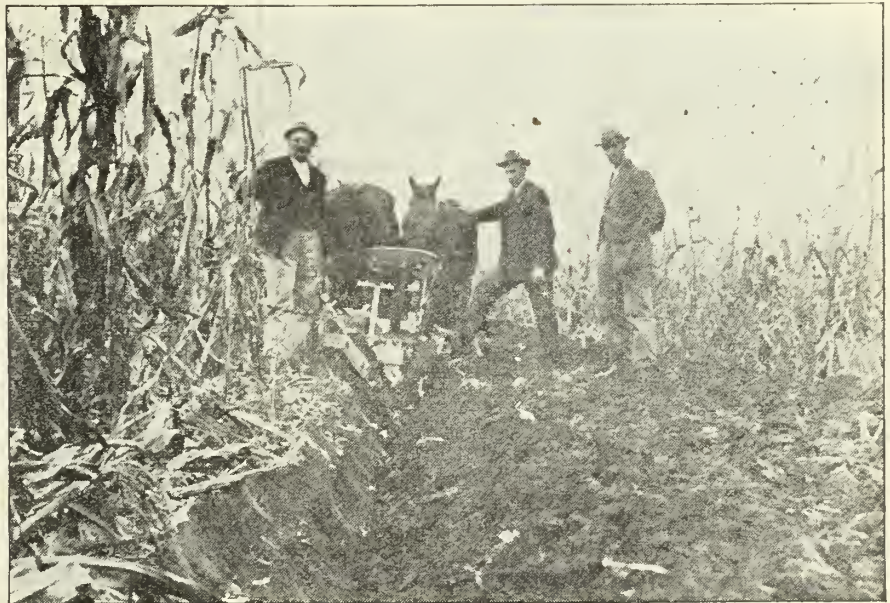
THE CORN STALKS ARE BURIED UNDER 12 TO 16 INCHES OF SOIL. SO DEEP THAT NEITHER DRILL OR HARROW CAN REACH THEM.
