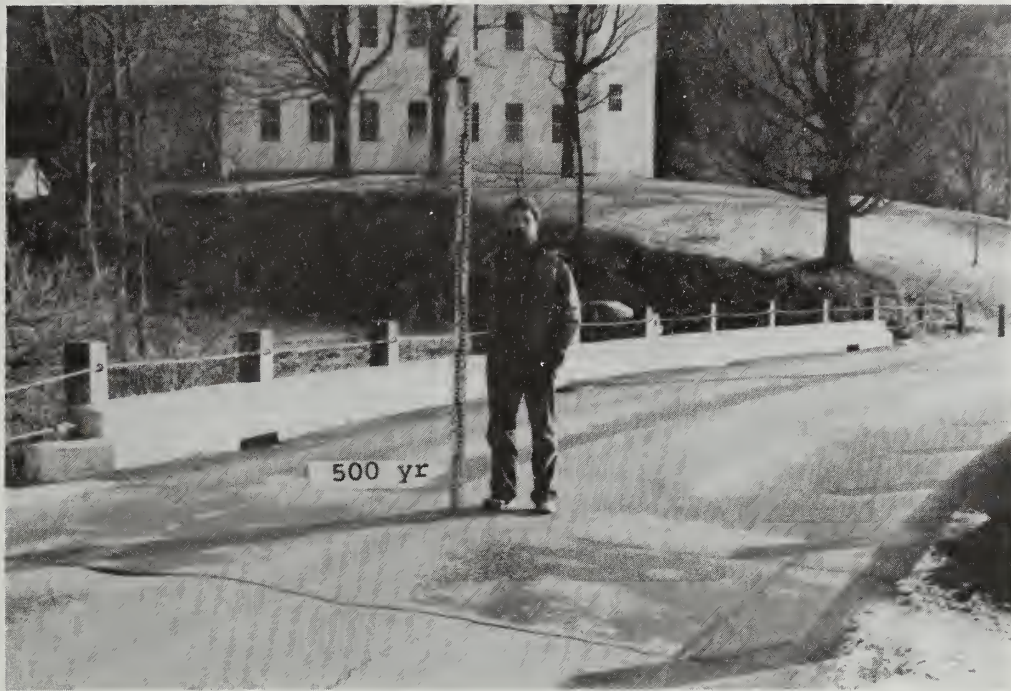
Figure 1. Bridge in Strafford over the West Branch of the Ompompanoosuc River at section WB14
