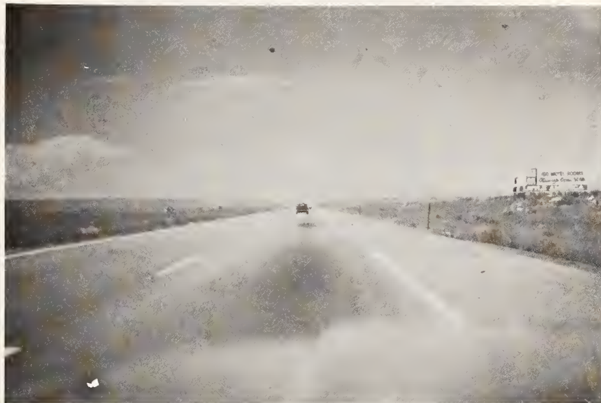
Figure B.22. Low Severity Depression (identified by oil droppings on pavement surface).
