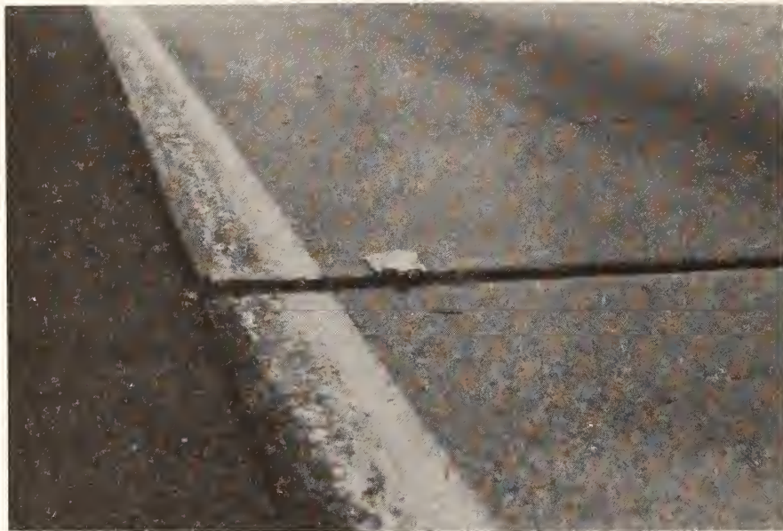
Figure C.11. Joint Faulting.
