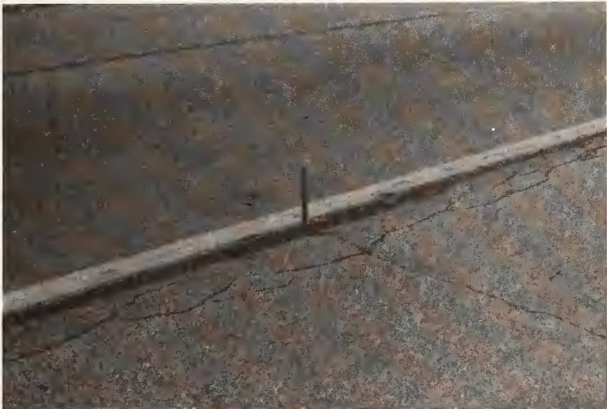
Figure C.19. Lane/Shoulder Dropoff.
