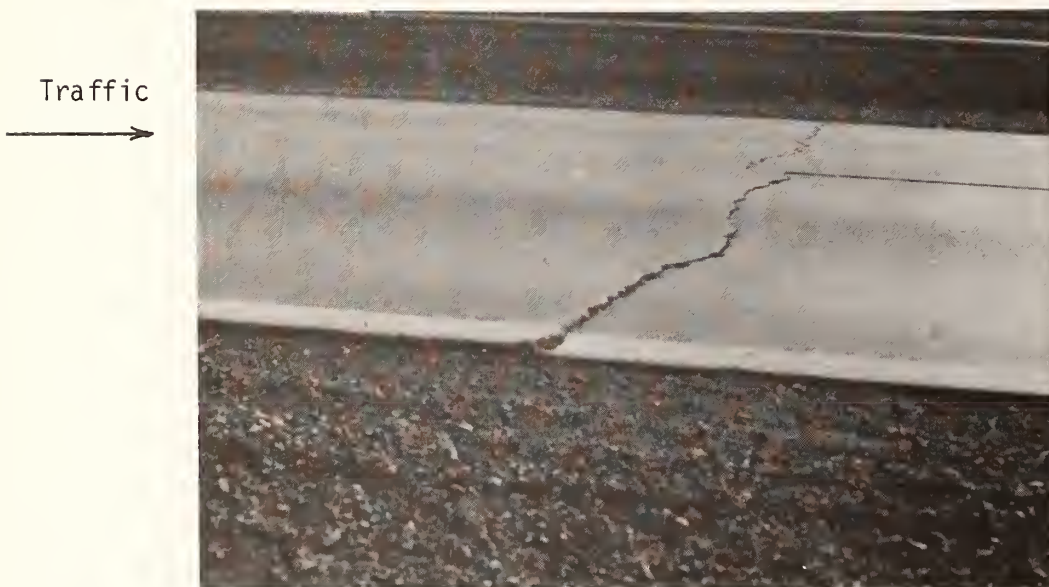
Figure C.10. Crack Faulting.
