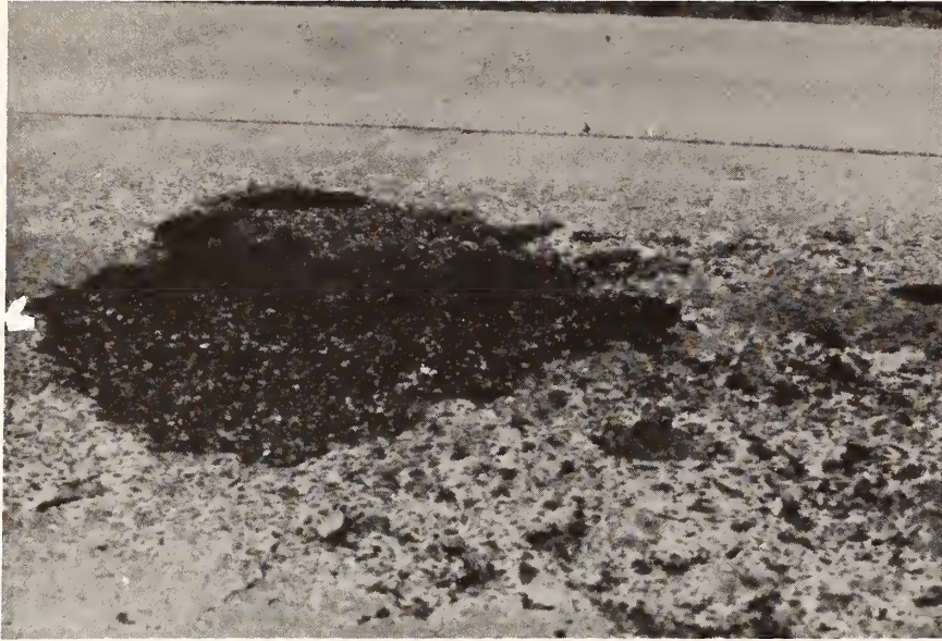
Figure C.41. . Scaling
