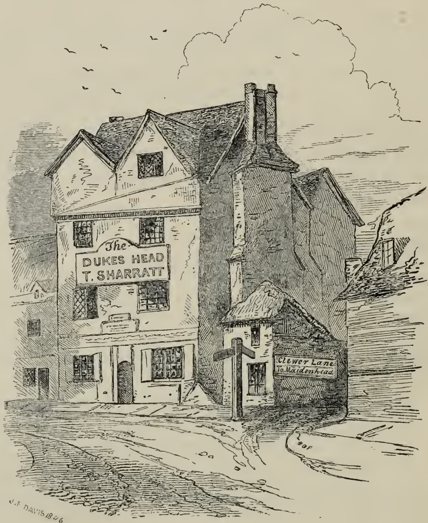
Old House at the lower end of Peascod Street.
