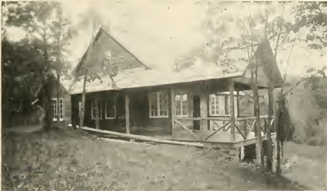
Another exterior on page 112, plan above J. Acker Hays, architect The joints of the prepared roofing are covered with a rubber preparation. From this side of the Sadler bungalow there is a magnificent view over the valley with the Hudson River in the distance
