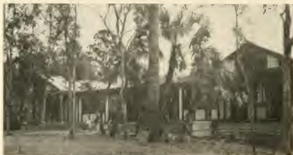
Plan on page 77 H. C. & H. F. Huntwell architects The Putnam bungalow was built in sections in New York City and shipped to Ormond Beach, Fla., where it was erected
