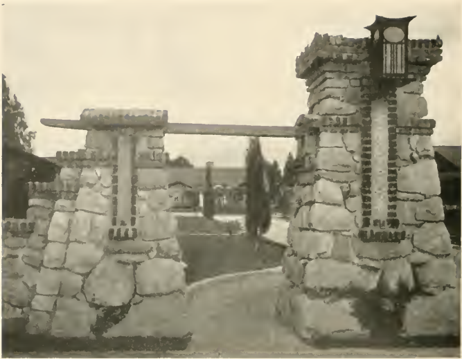
Plan on page 77; individual bungalows on pages 14, 21-25, 130, 132 Sylvanus Marston, architect The footpath entrance to St. Francis Court, Pasadena—a striking instance of the very common use throughout Southern California of rough clinker brick in conjunction with stone work
