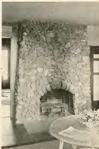
A rather unusual type where very rough stone is used throughout the chimney breast, and the mantel is omitted entirely
