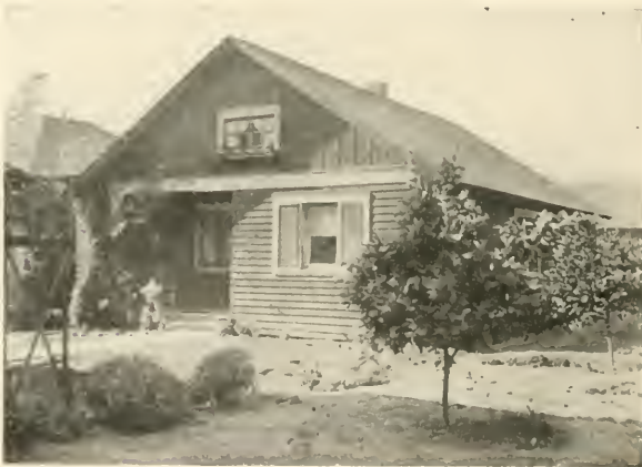
Clapboards differ but slightly in appearance from the overlapped boards, but they are narrower. The cost was $700
