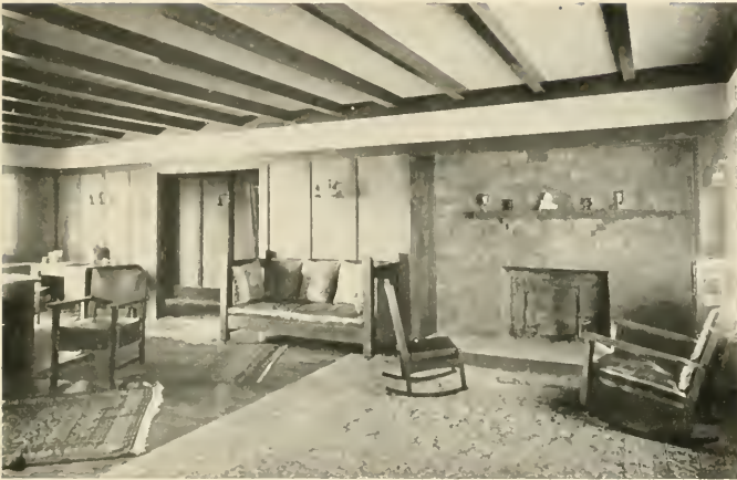
Exteriors on pages 57, 114, 115; other interior on page 151 — George A. Clark & L. du P. Millar, architects In the Childs California home the recessed fireplace is faced with brick set on edge instead of on their sides, as ordinarily found. Usually a flat arch will be found more attractive over the opening, instead of supporting a regular course of bricks or an iron bar as here. The heavy shelf of a redwood beam is supported by corbeling
