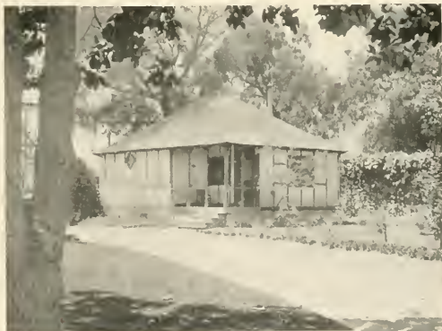
Another example of the tent-house type of summer home. There has been an effort at decorating the canvas by painting under the shelter of the porch
