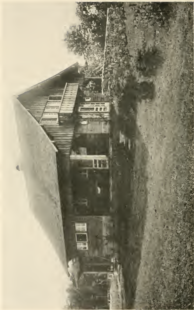
The summer home of Mr. J. B. Strongman, Westboro, Mass., an adaptation of the Swiss chalet. The walls are of unplanned boards, battened on the inside for the lower part and on the outside for the upper story
