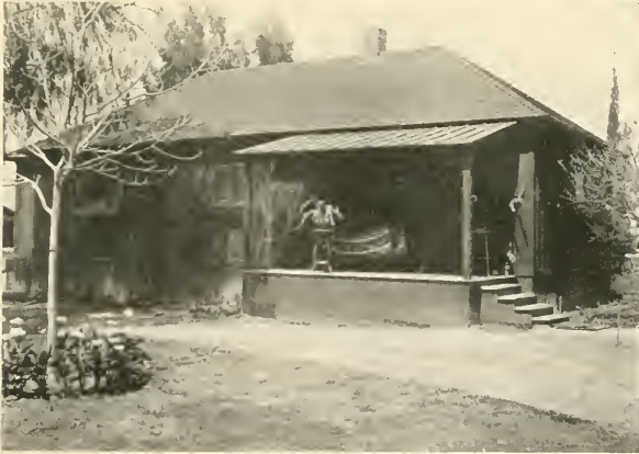
The foundation here is of rough redwood boards, set an inch or two apart with battens on the inside
