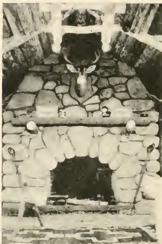
A very good piece of arch work with large stones and raked-out joints. Notice the shelf of a half-log supported on log pins
