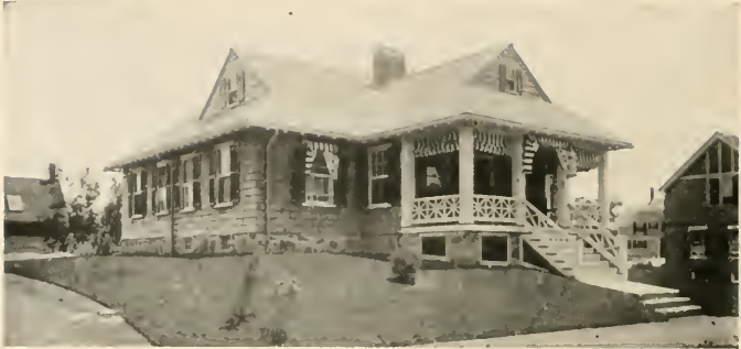
A continuous wall of stone has been used, with a raised line of pointing on the outside. The latter would be out of place with a less finished style of summer home
