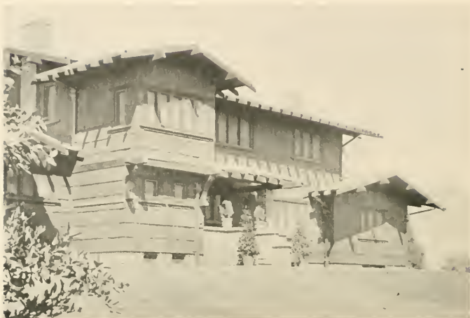
Other exteriors on pages 117, 118; interiors on pages 145, 151. Geo. A. Clark & J. du P. Millar, architects The roof of the Childs California home is covered with one of the prepared roofings that comes in a dull lead color
