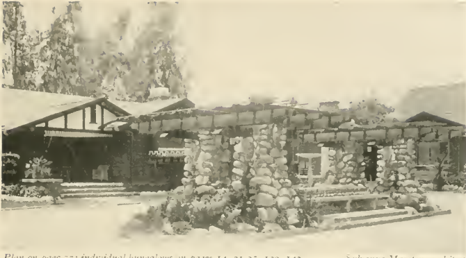
Plan on page 77; individual bungalows on pages 14, 21-25, 130, 142 Sylvanus Marston, architect At the near end of the Court the driveway turns around a fountain which is a very popular gathering place in the late afternoons
