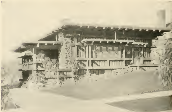
A Western Coast bungalow that displays a remarkably daring utilization of modified Japanese motives. The roof, it will be noticed, is almost flat. The walls are made up of whole timbers
