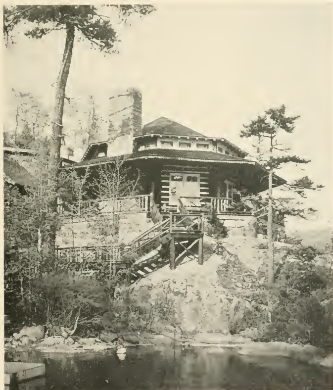
Exterior of No. 100, 117-119; interior of the Log Cabin, both designed by M. Grath & Shepard, architects The typical Adirondack lodge, this particular example being on Lake Wilbert, Franklin County, N. Y. The structure is of smooth logs with plastered chinks
