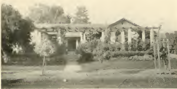
Plan below Francis W. Wilson, architect Mr. Wilson's bungalow is doubly enjoyable in that it has, in addition to the patio in the rear, a still larger space in the front sheltered by the vine-covered pergola motive
