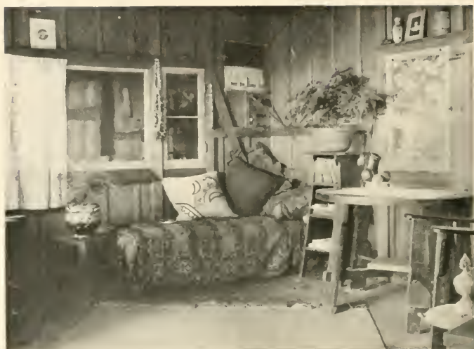
An inside finish of batted boards is used here, giving the effect of being set back so as to leave the studding frame slightly projecting
