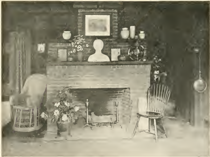
It is easier to construct a fireplace of brick throughout, and usually more pleasing where the room is small—a stone fireplace shows to best advantage in a very large room
