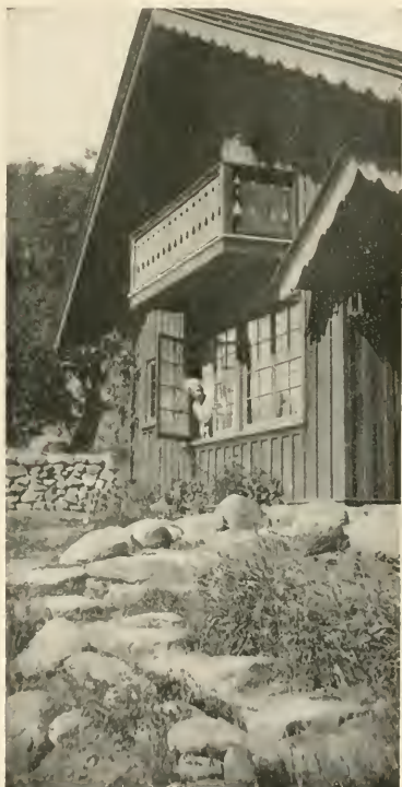
See also Frontispiece and pp. 40, 57. Myron Hunt & Eimer Gray, architects The characteristic ornament of the Swiss chalet type—sawed-out eaves boards and balcony railing
