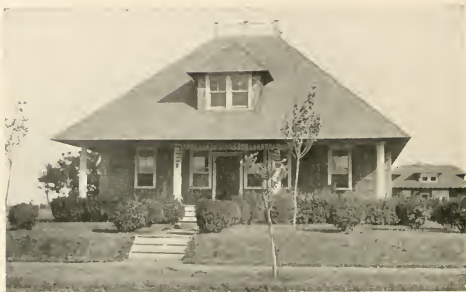
When the plan approximates a square this type of roof will probably result, although where there is no second story the pitch will be much lower and the dormer will be omitted to preserve the true bungalow character
