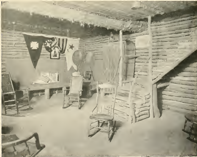
A rustic interior finish such as this is not often seen, which is just as well, perhaps, for its untidiness is hardly offset by intrinsic beauty. It is a difficult matter to carry rustic work, either inside or out, to a point short of affectation
