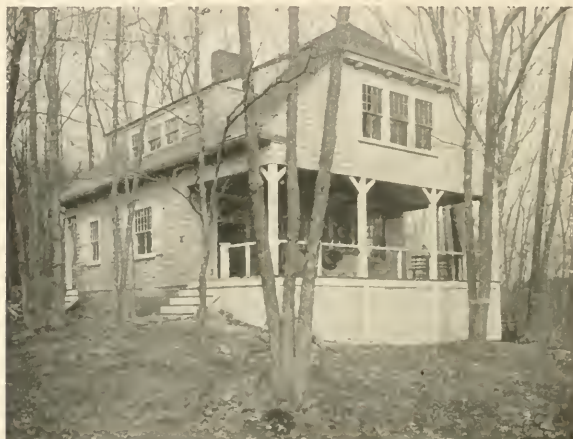
Plan on page 77, interior on page 100, No. 130 William P. Hubon, architect Mr. Hubon's camp near Salem, is said to have been built at a cost of $1100, of shingles that have been allowed to weather
