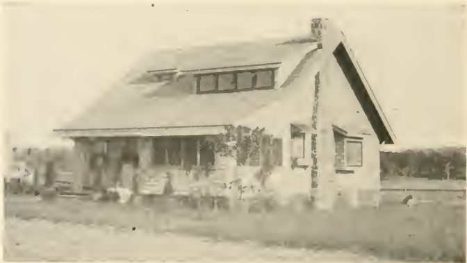
Brick piers are used here, with stone for the chimney. Whatever piers are used, latticework should close the openings between them
