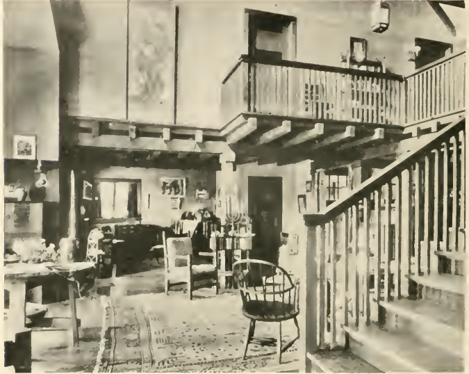
An interesting effect has been secured by leaving the floor joists uncovered to form the ceiling of the first story. The balcony is supported on these floor joists as cantilevers
