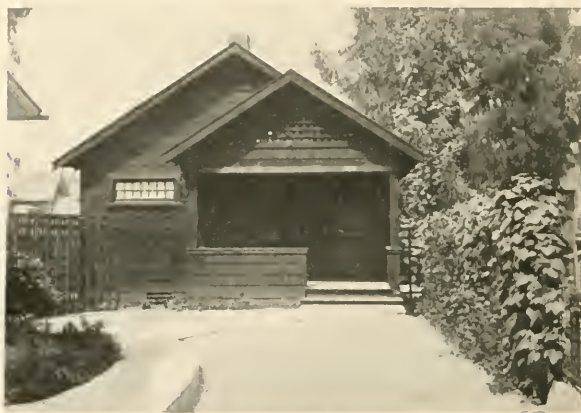
The side walls of shakes are carried directly down to the ground—a rather unusual form of foundation excepting in cheap construction. This whole bungalow cost but $1200. It consists of five rooms and a bath
