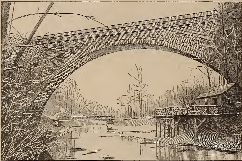
CABIN JOHN BRIDGE The longest stone arch in America, located near Washington, D. C. Through the conduit inclosed by this bridge passes all the water-supply of the national capital
