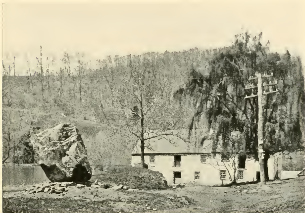
GULPH MILL. Erected 1747
