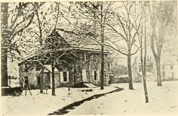
HESTON HOMESTEAD Built 1766. Torn down 1877
