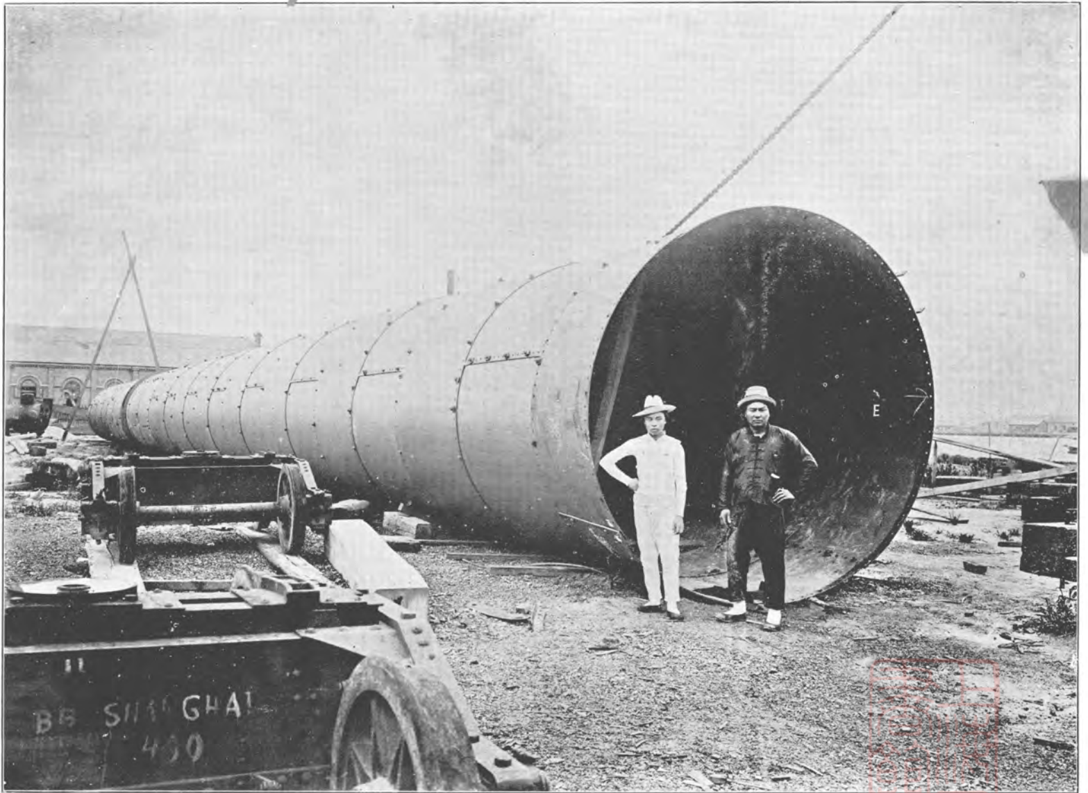
Steel Chimney, built and erected for Hupeh Cement Factory, Dimensions 200 ft long, 15 ft, diam, Weight 55 tons. (1)
