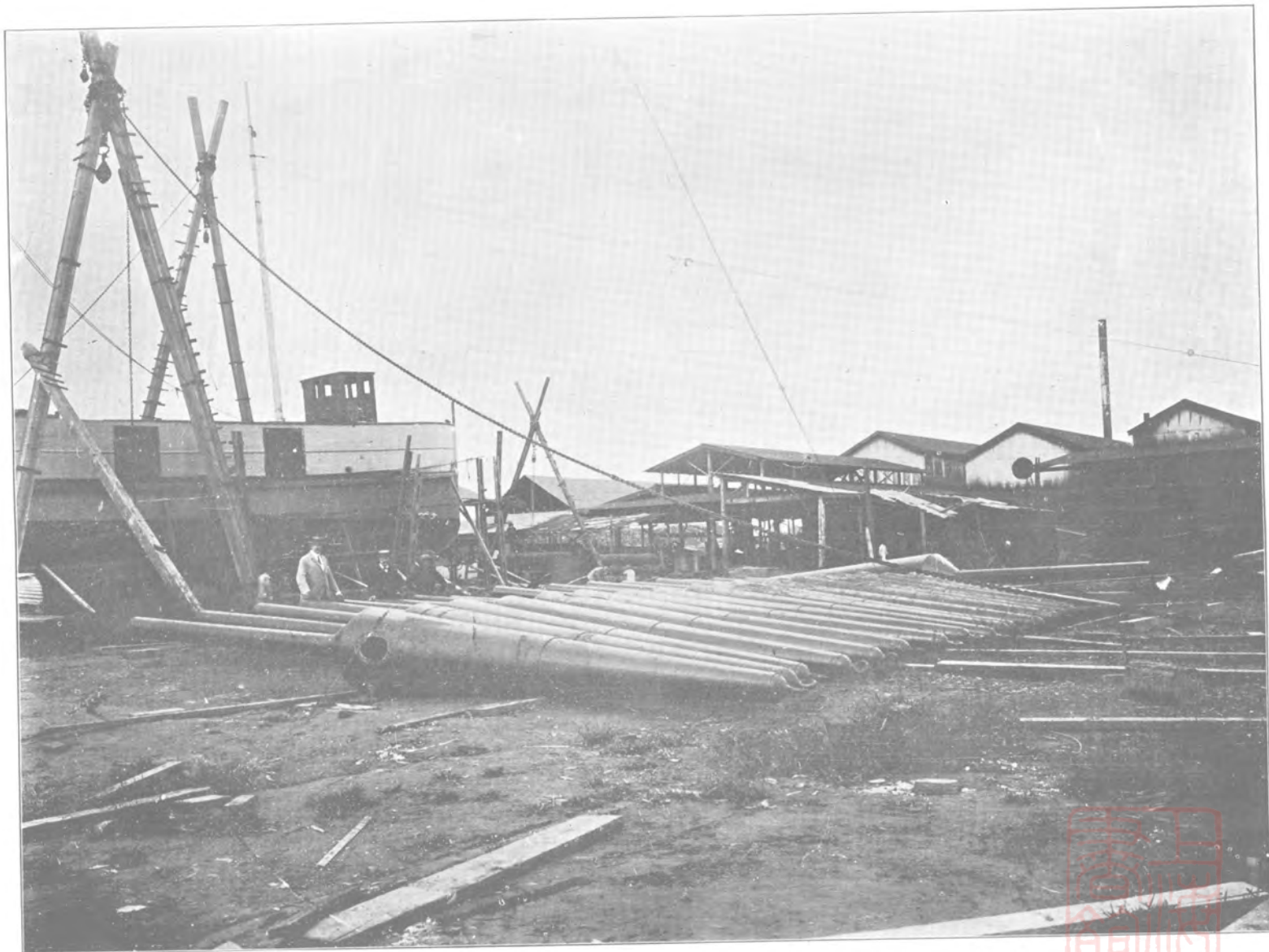
A Lot of Steel Spar Buoys, built for Chinese Imperial Maritime Customs, Shanghai, Dimensions 30'0" long \times 3'0" diameter, Weight \frac{1}{2} ton,
