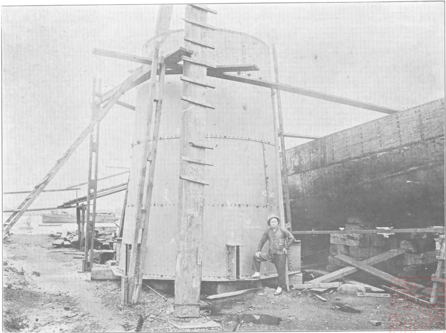
The Lower Part of Chimney (2)
