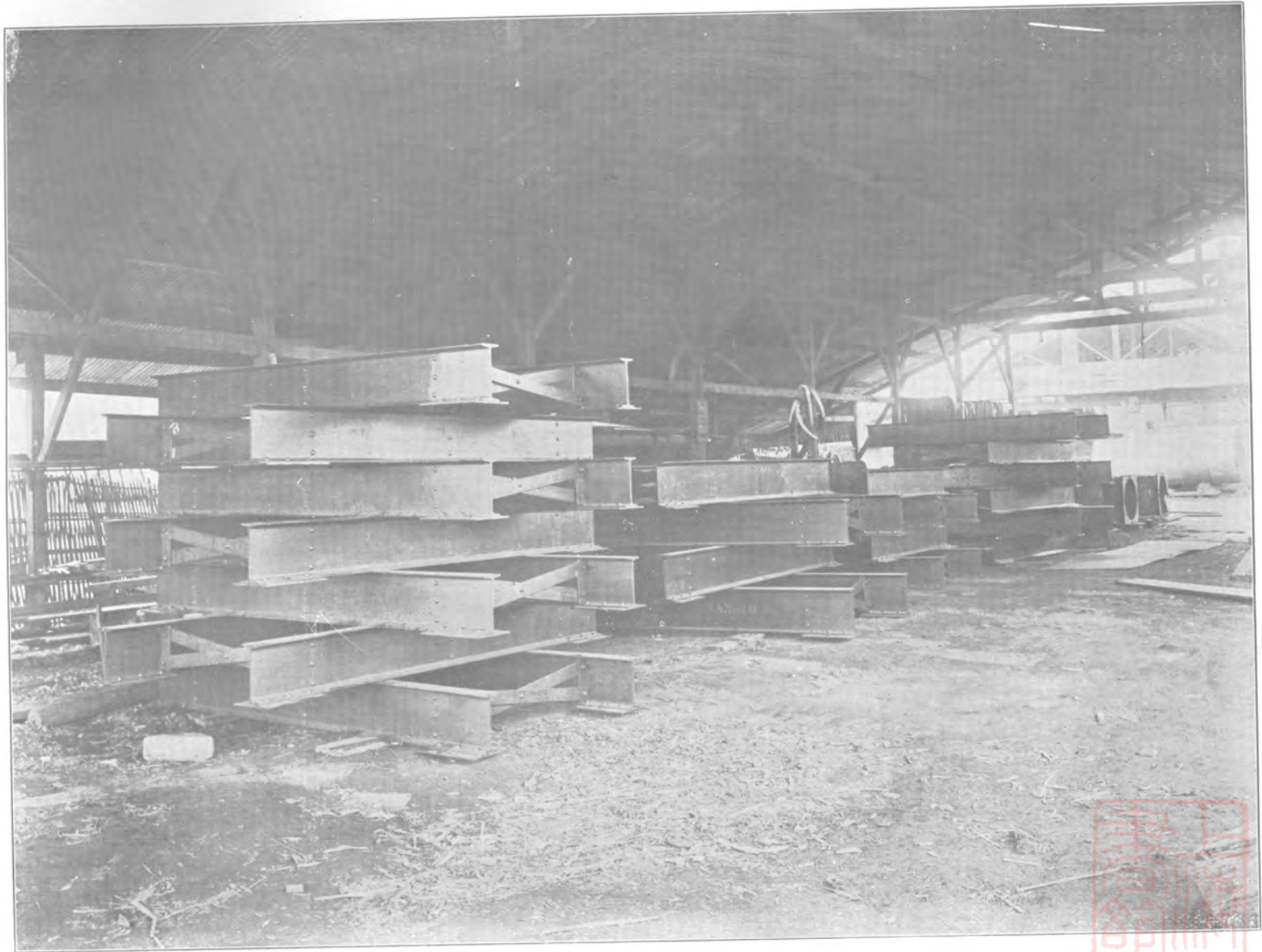
Small Steel Girders, built for Chekiang Railway Co.
