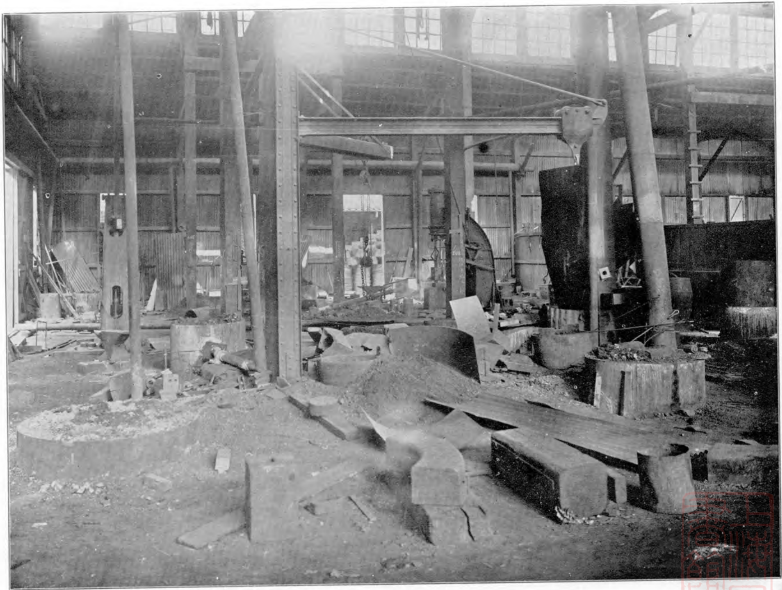
View of Blacksmiths' Shop
