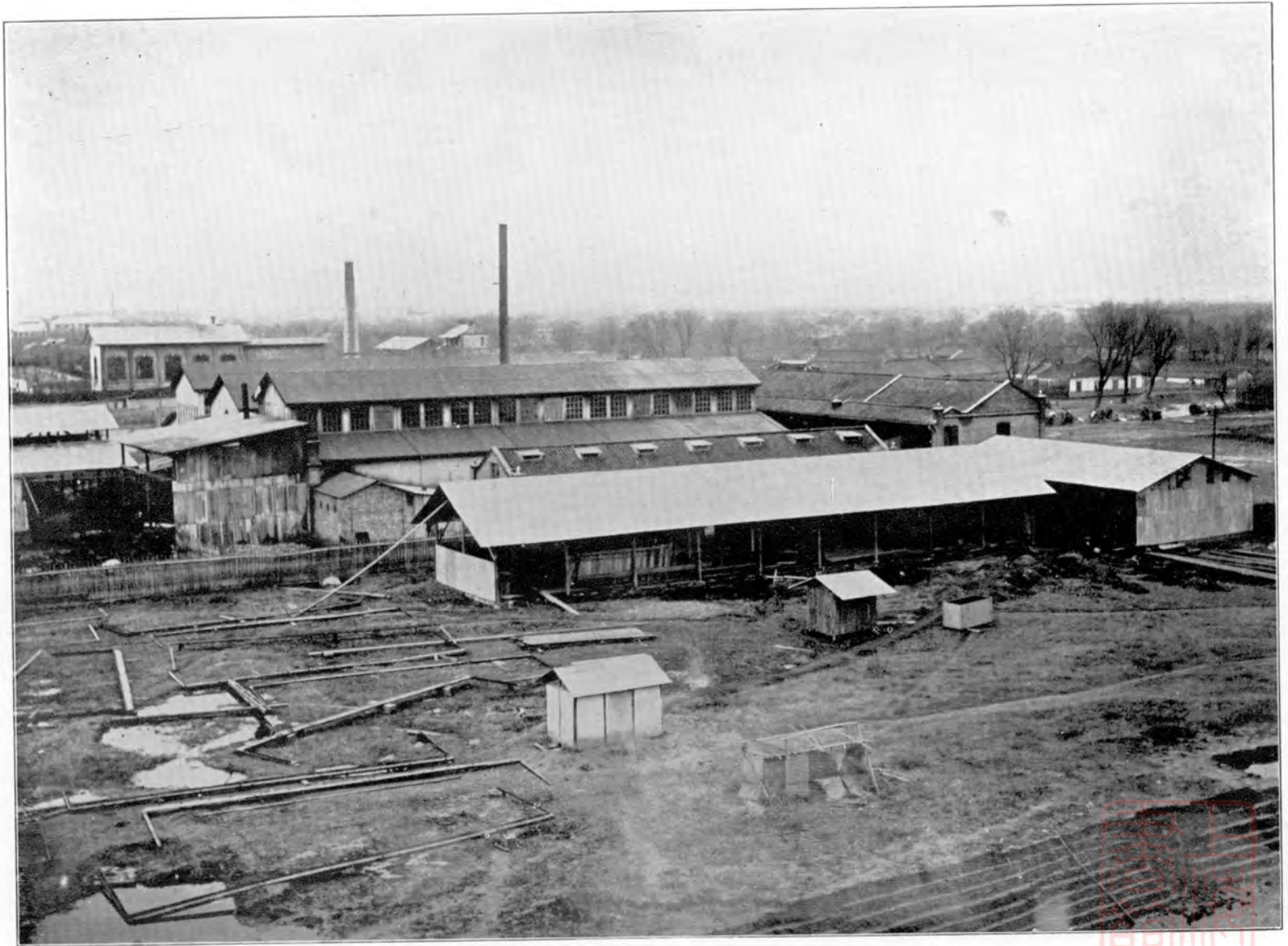
View of Whole Works
