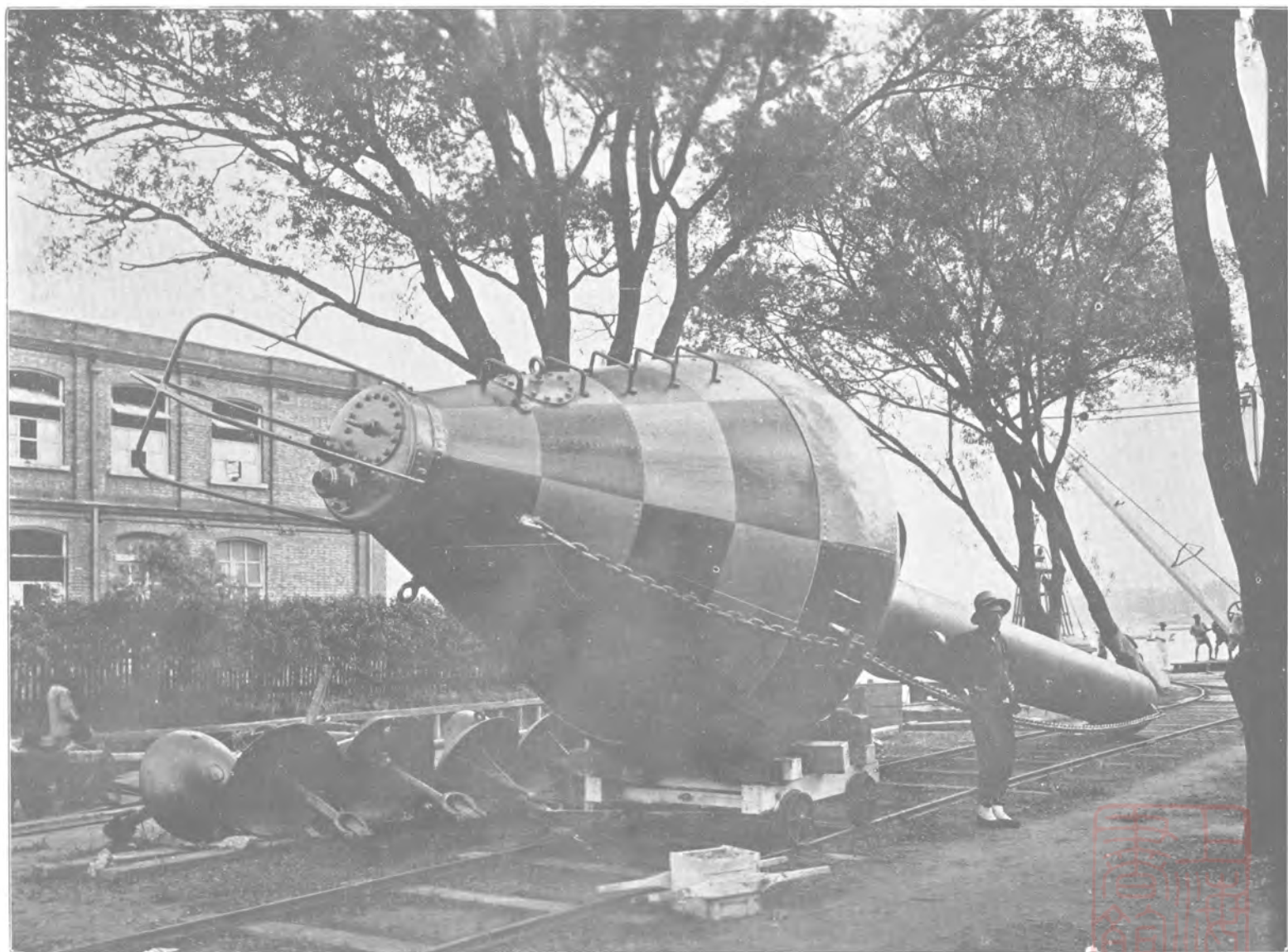
View of an Automatic Whistling Buoy, built for Chinese Imperial Maritime Customs, Shanghai.
