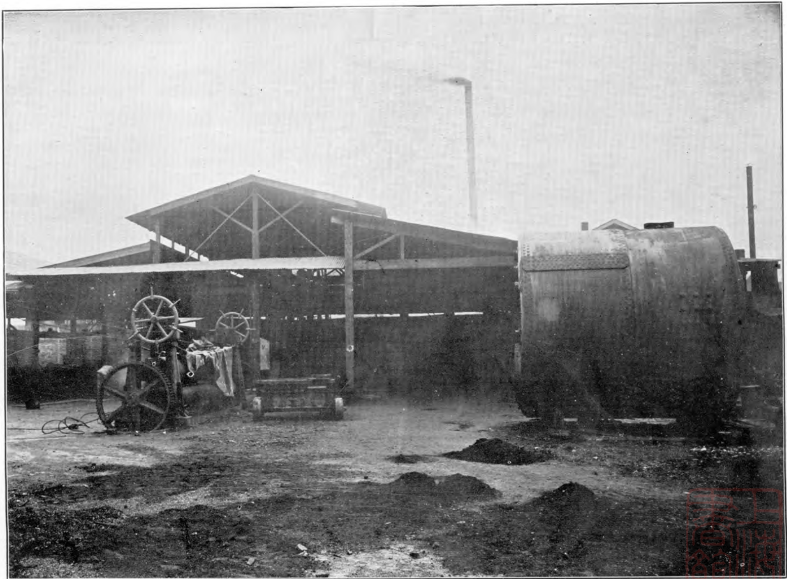
View of Boiler Makers' Shop
