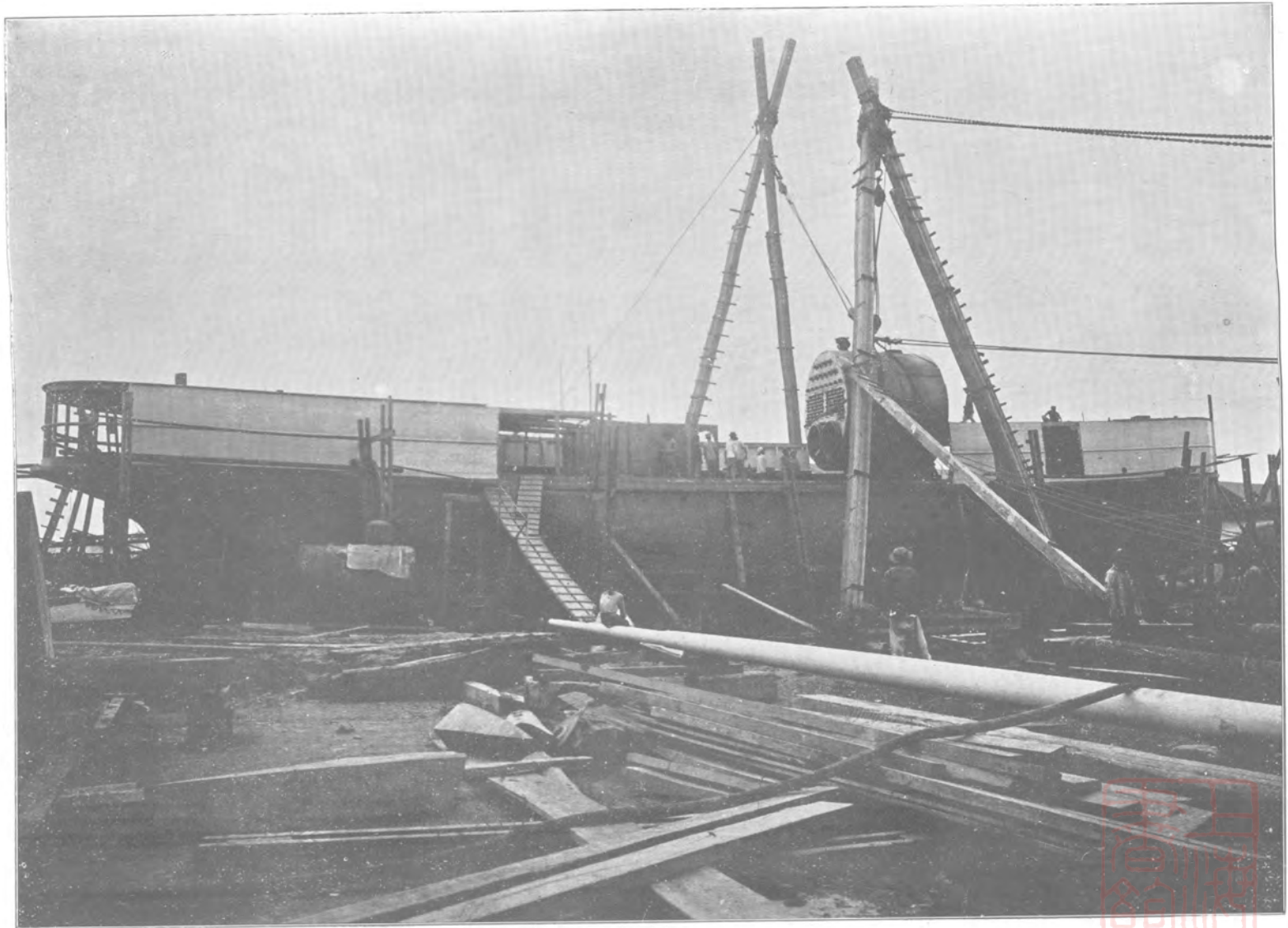
Lifting on board Boiler, weighing 23 tons
