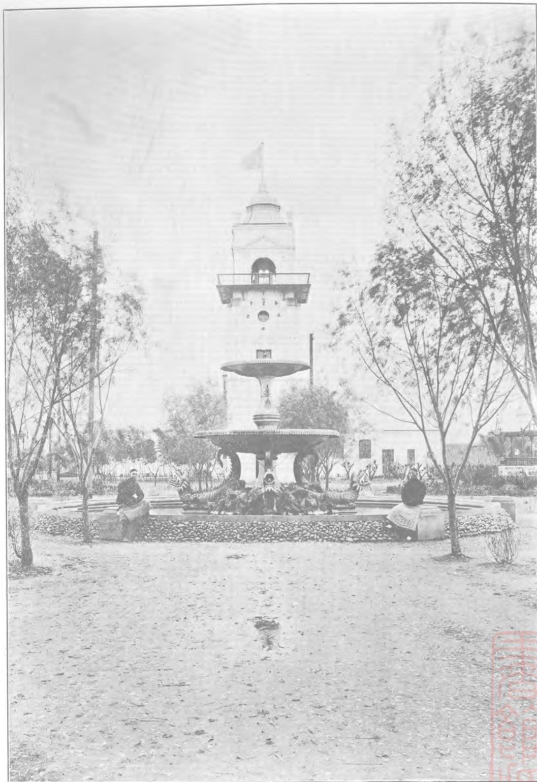
View of a cast iron Ornamental Fountain, built and erected for Nanking Exhibition, 1910.
