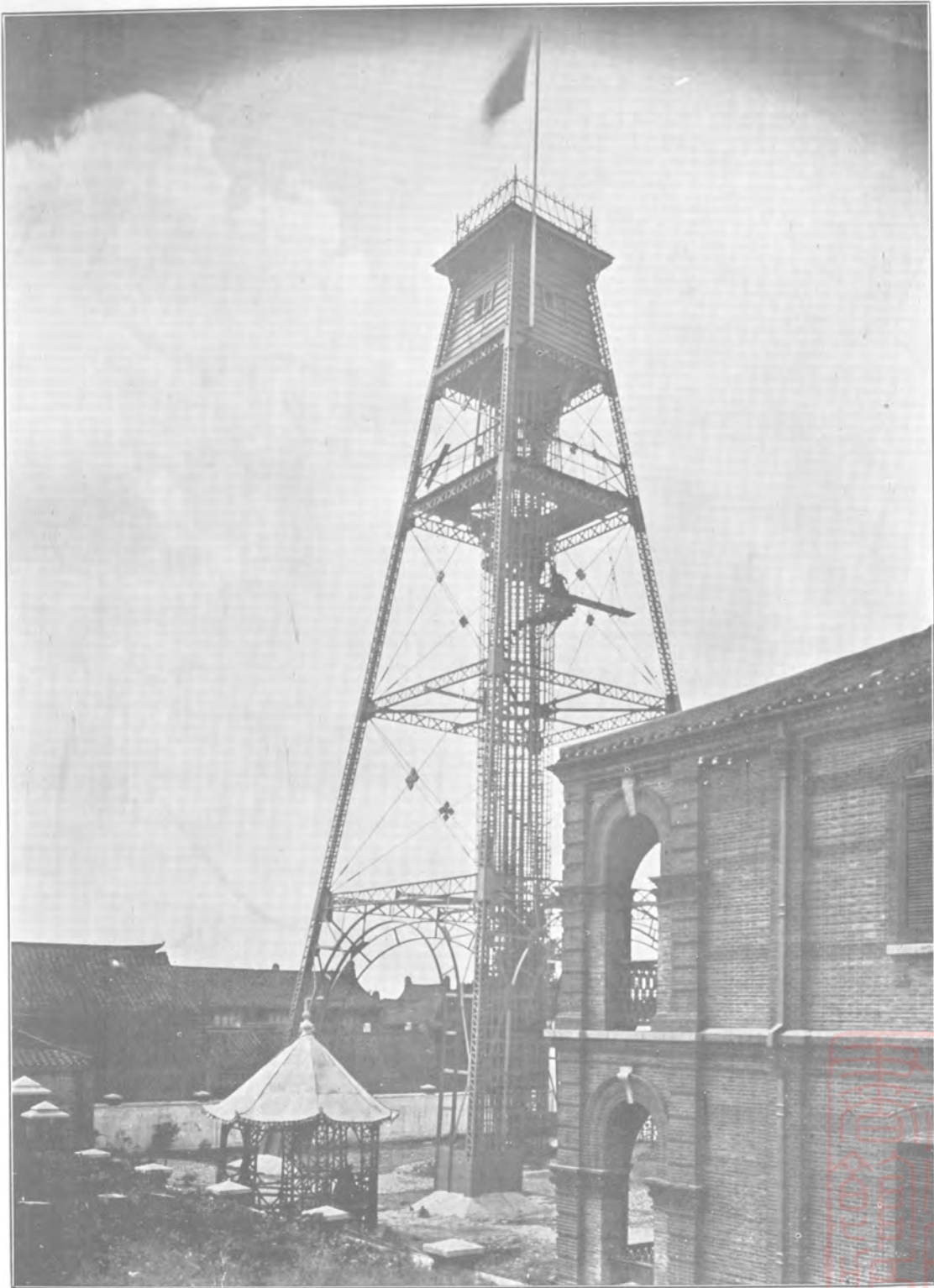
Steel Watch Tower with Alarm Bell, built for Chinese City, Shanghai, 129-2 Height 110 ft, complete with one Brass Bell, weighing about 6000 lbs.
