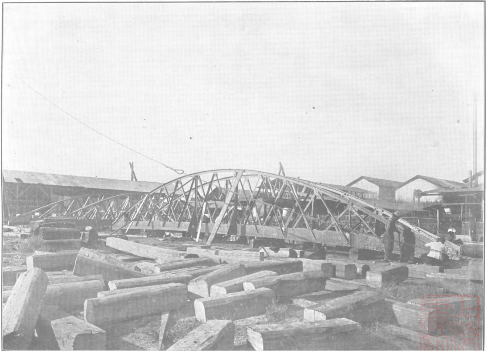
Steel Bridge "Yuen Chung", 200' 0" long (in 3 spans) for Ningpo.
