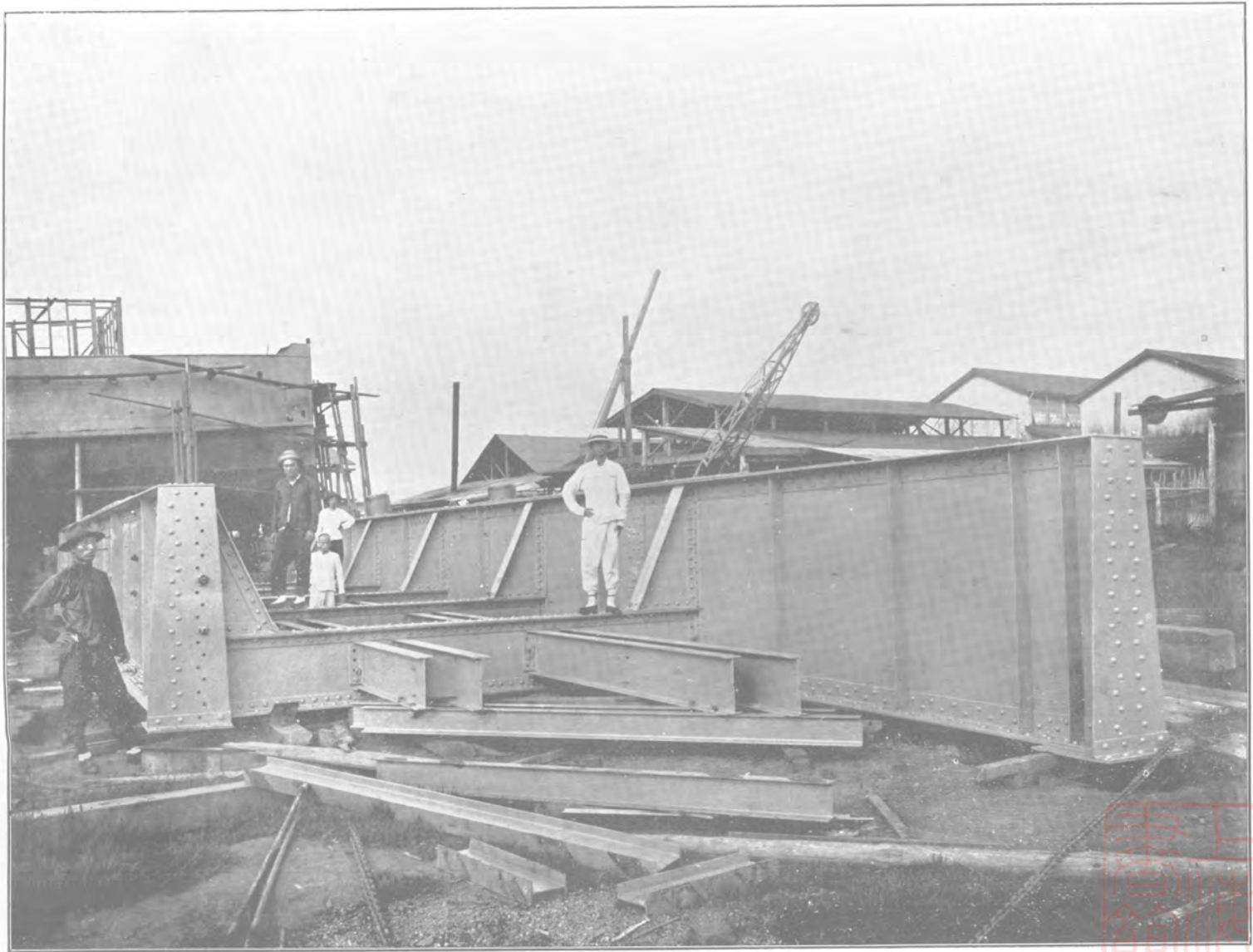
Skew Steel Rrilway Bridge, built for Kiangsu Railway Co. Dimensions: length 65 ft, width 15 ft, height of plate girder 6 ft, Weight 38 tons, Carrying Load 5000 lbs per sq. ft
