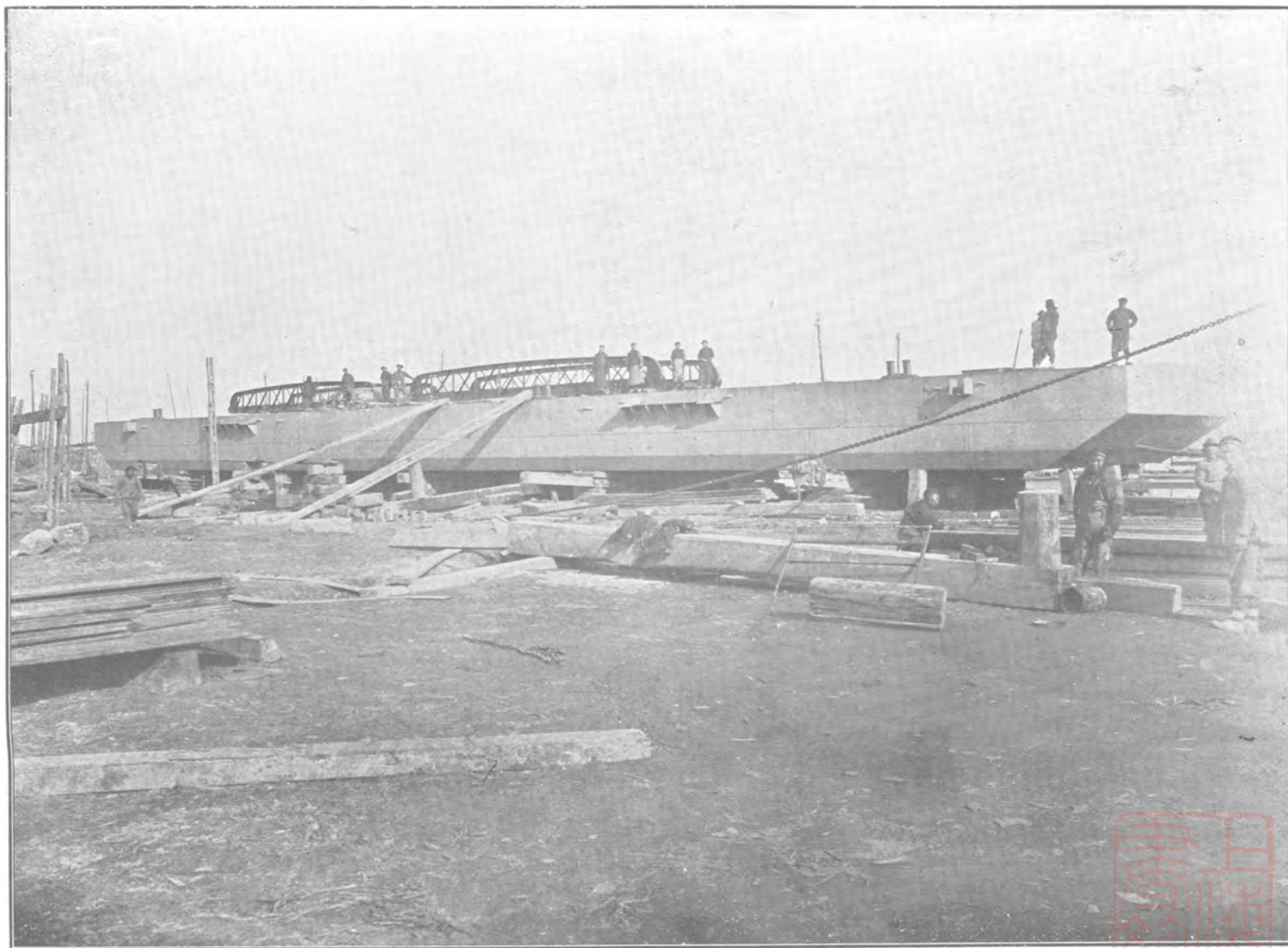
Steel Pontoon, built for Kiangnan Arsenal, Dimensions 160'0" long, 27'0" wide 8'0" deep
