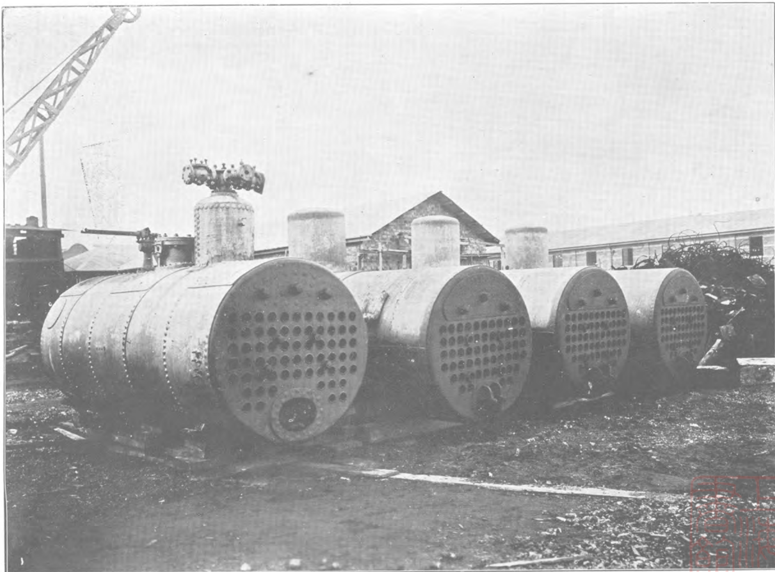
Multitubular Underfired Boilers, 18' long \times 5'6" diam, 120 lbs W. P., for Engine of 100, H. P.
