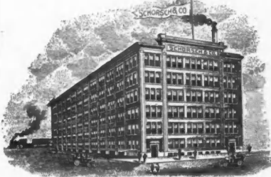
FACTORY 132 ND TO 133 RD ST. & BROOK AVE.
