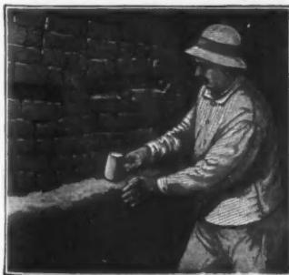
Showing ease with which Pilibrico is laid in place.
