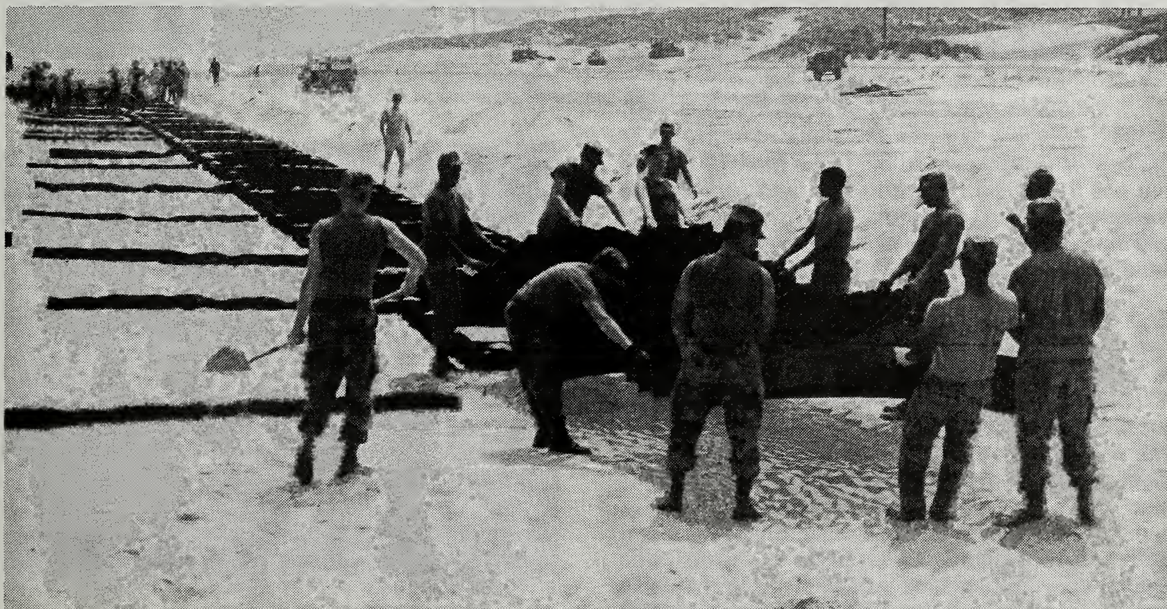
Figure 20. Using sand fill in cellular confinement system.
