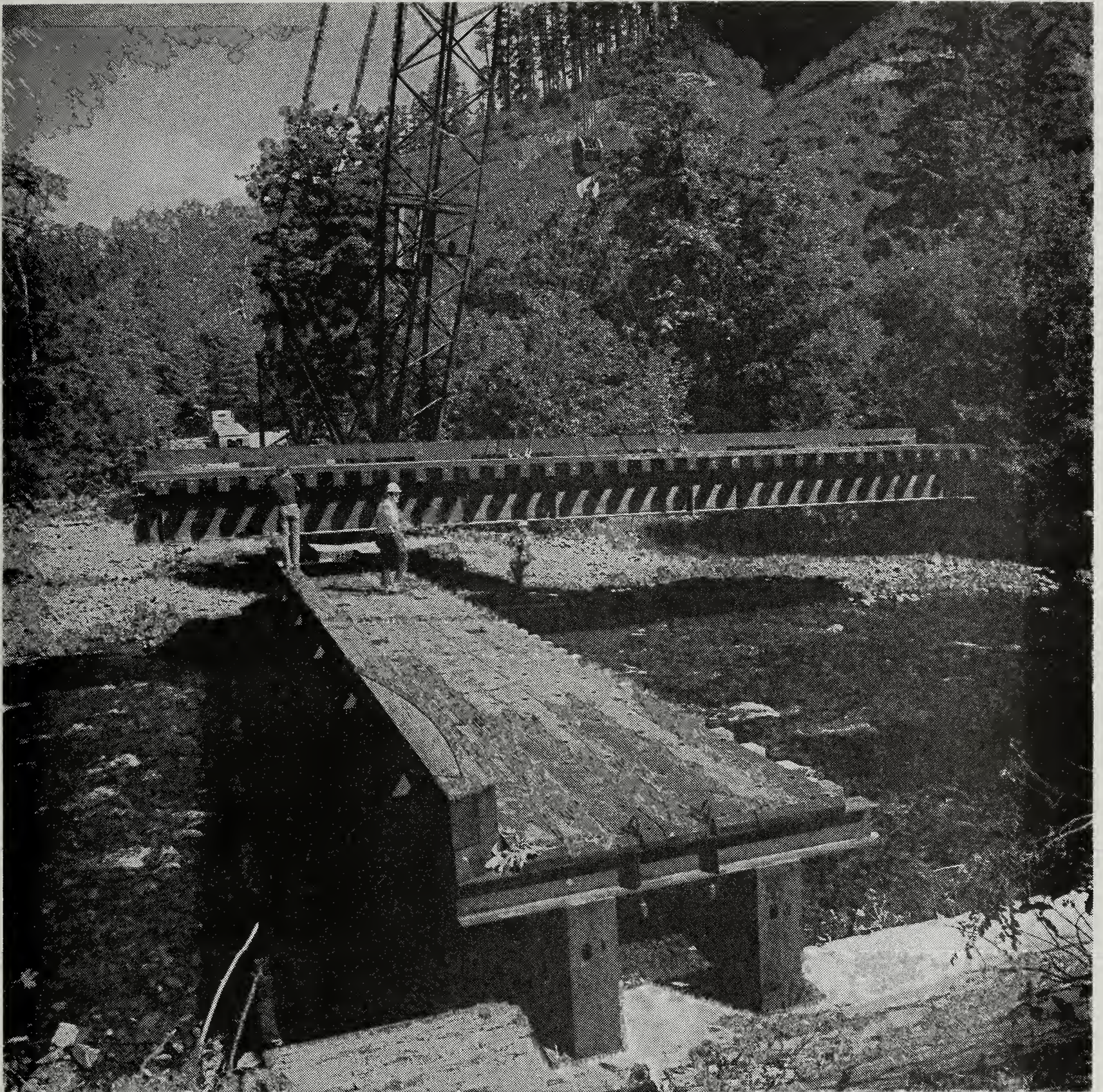
Figure 43. Prefabricated superstructures normally are lifted in place with a crane.
