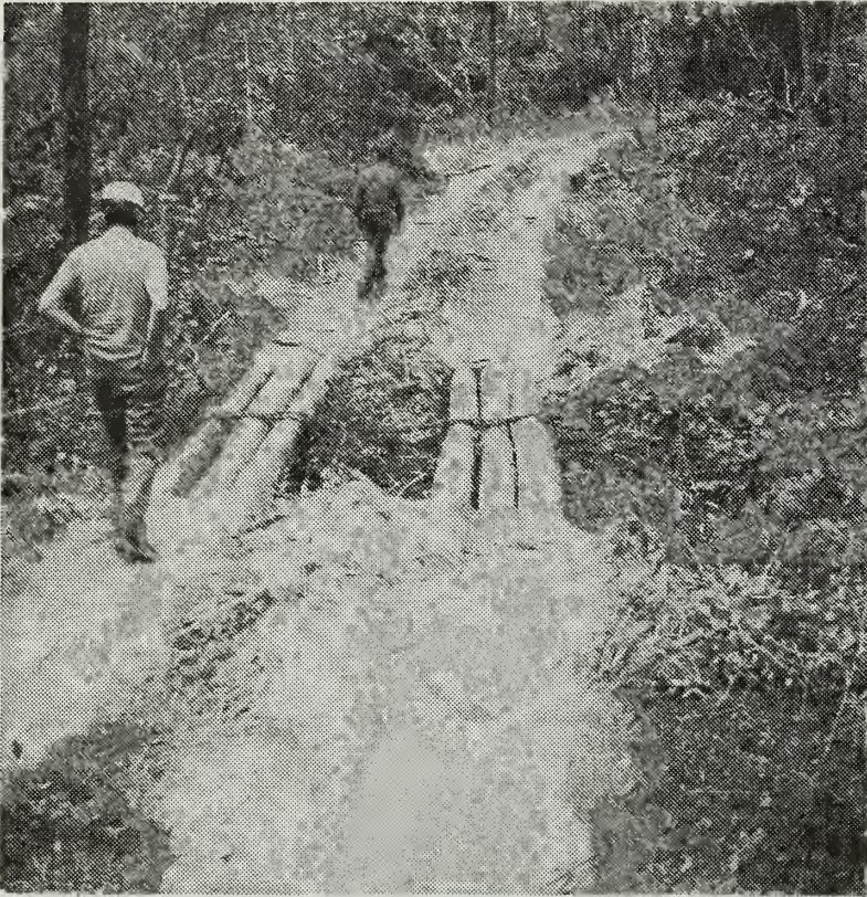
Figure 9. Logs, bound together, used as a crossing.
