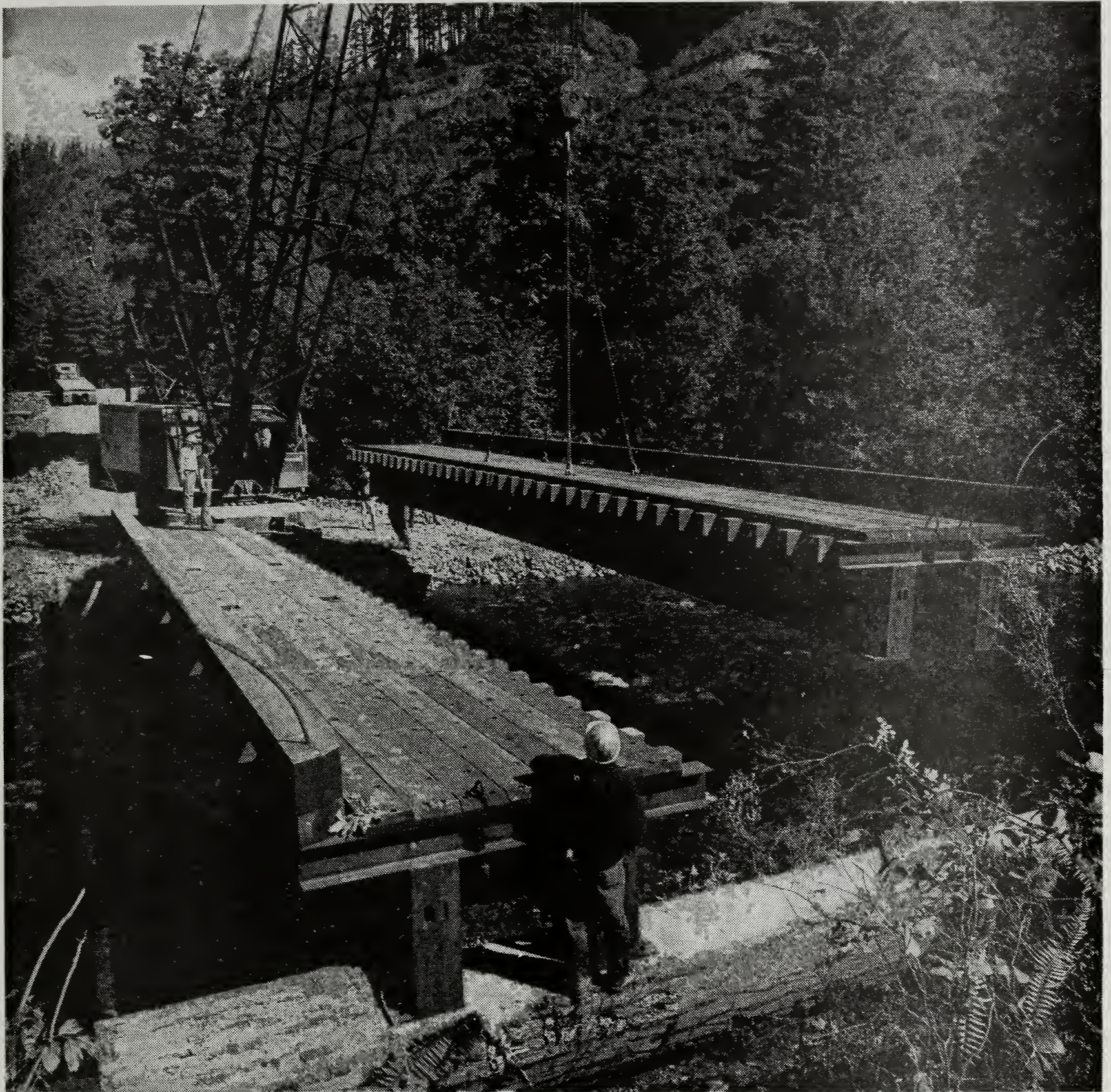
Figure 10. Installing a prefabricated bridge.
