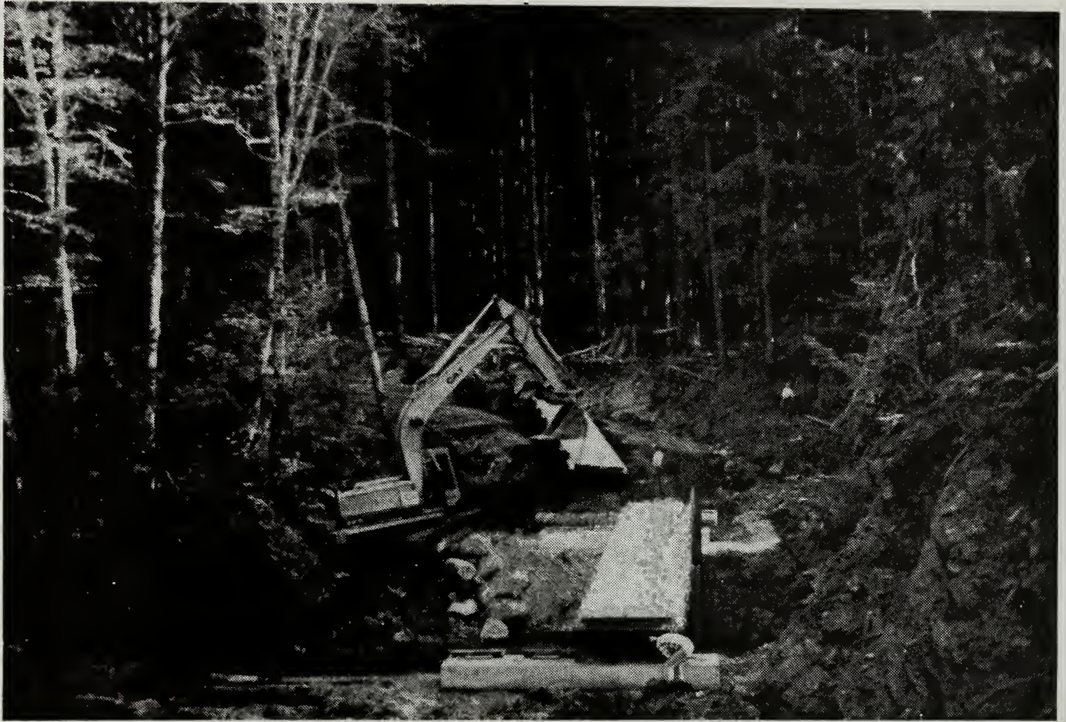
Figure 44. BIG R prefabricated bridge can be installed with logging equipment.
