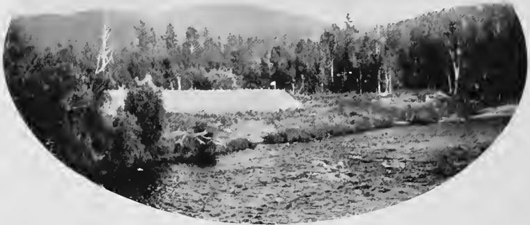
A break in the embankment in Trans-Baikalia.
