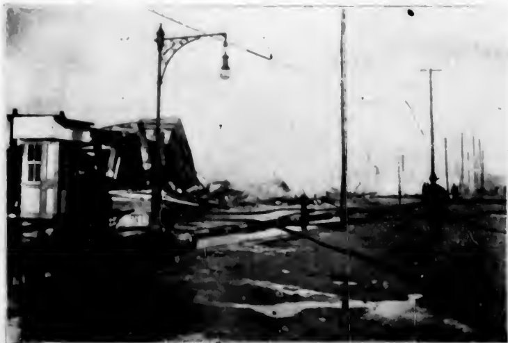
View looking west on Surf avenue. Ruins of the Whirlwind Ride at left.
