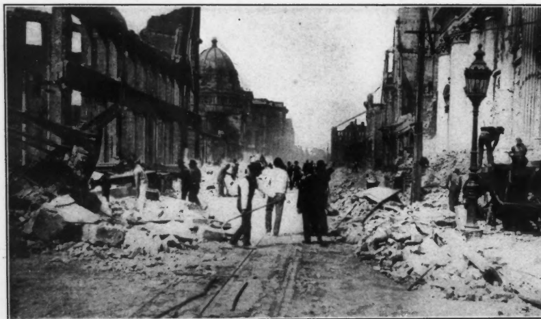
NO. 2. CLEARING A STREET.
