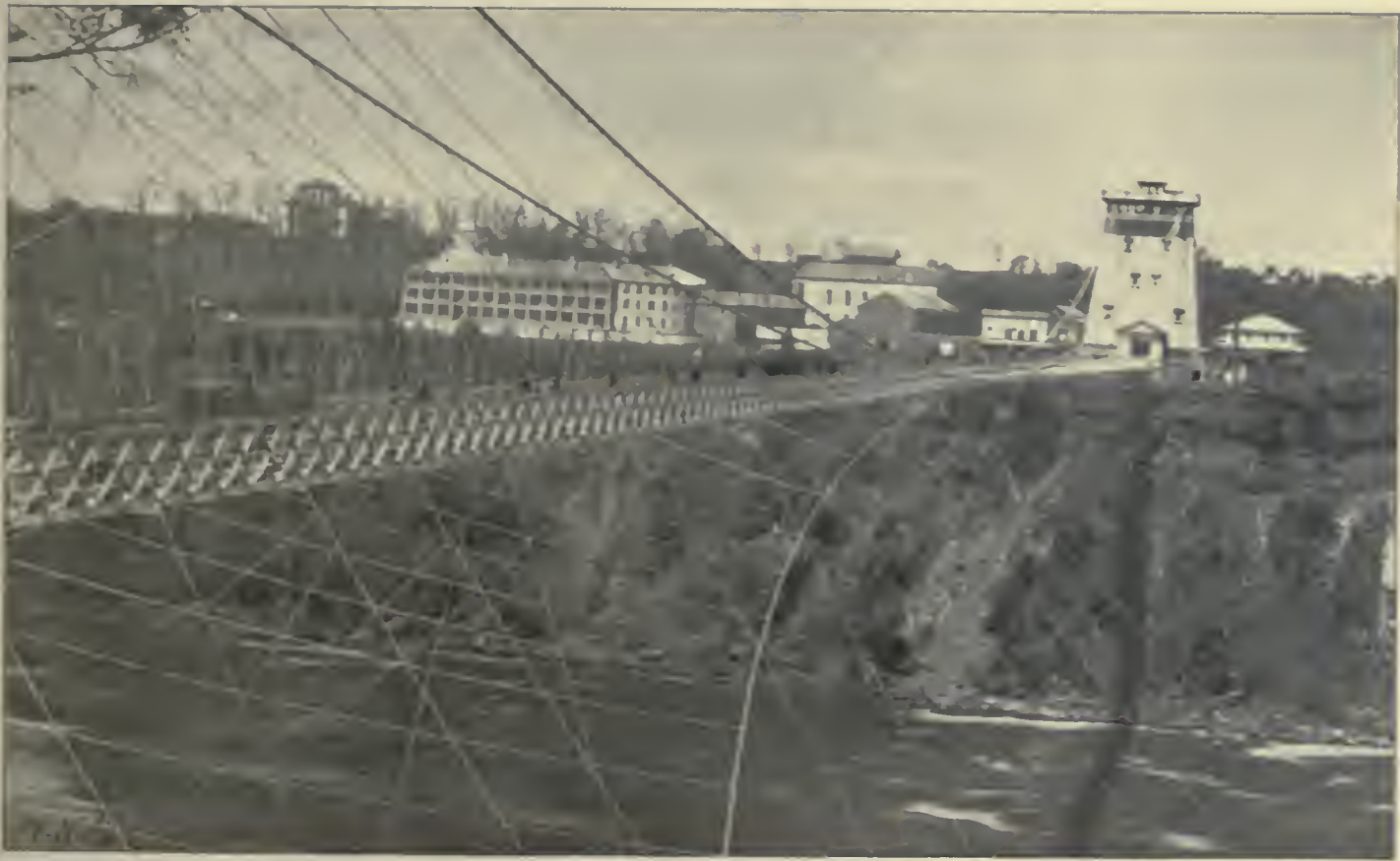
SUSPENSION FOOT AND CARRIAGE BRIDGE FROM BELOW STATE RESERVATION.
