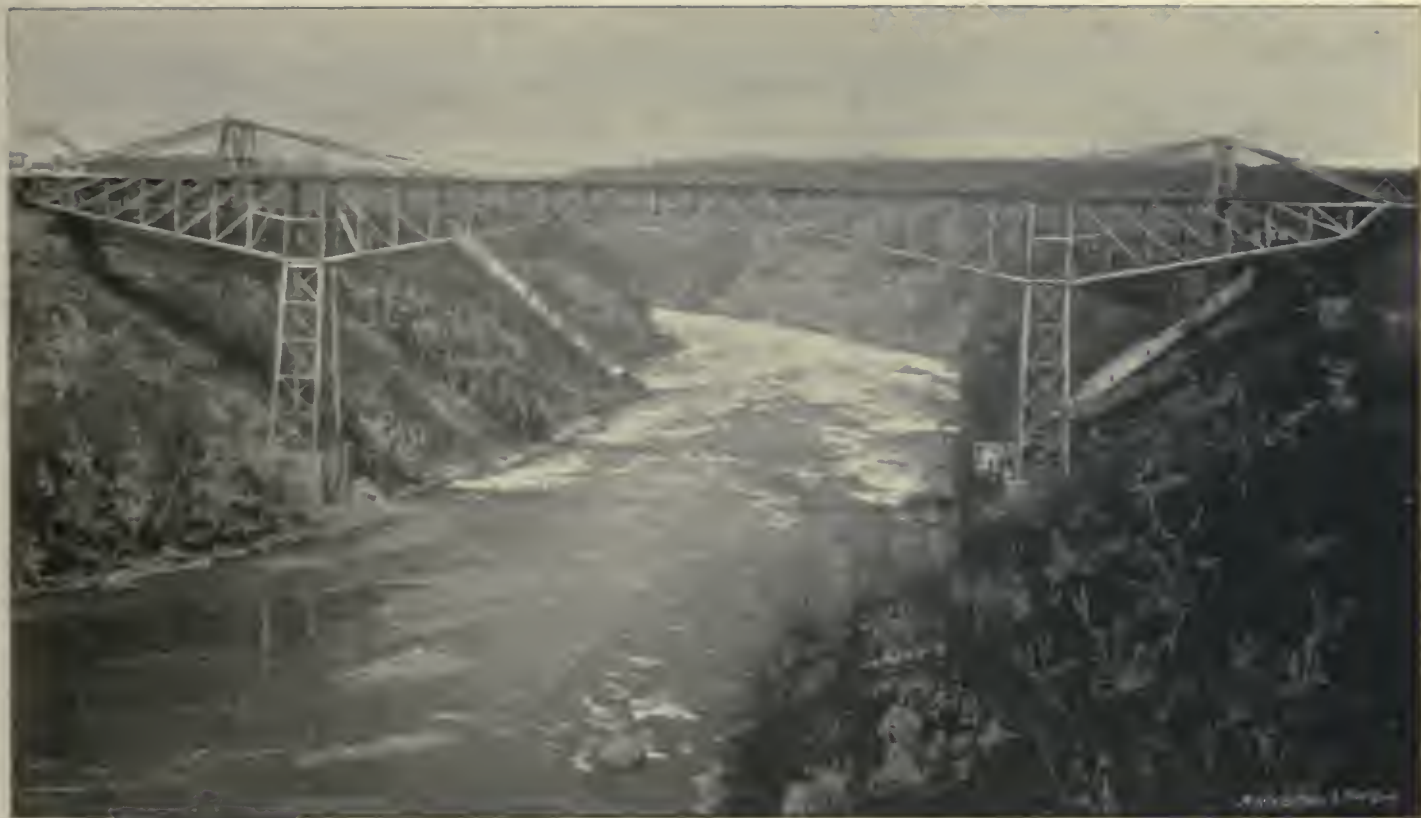
THE STEEL CANTILEVER BRIDGE OF THE MICHIGAN CENTRAL
