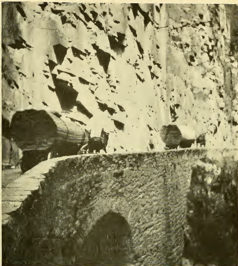
IN THE EGGEN-TAL: TIMBER WAGONS GOING DOWN FROM THE SAWMILLS INTO BOZEN
