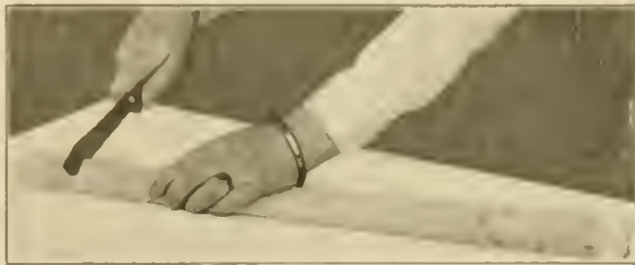
A sharp carving knife, a pair of pruning shears or an old-fashioned hay cutter (if you live on a farm) will cut the rolls easily.
