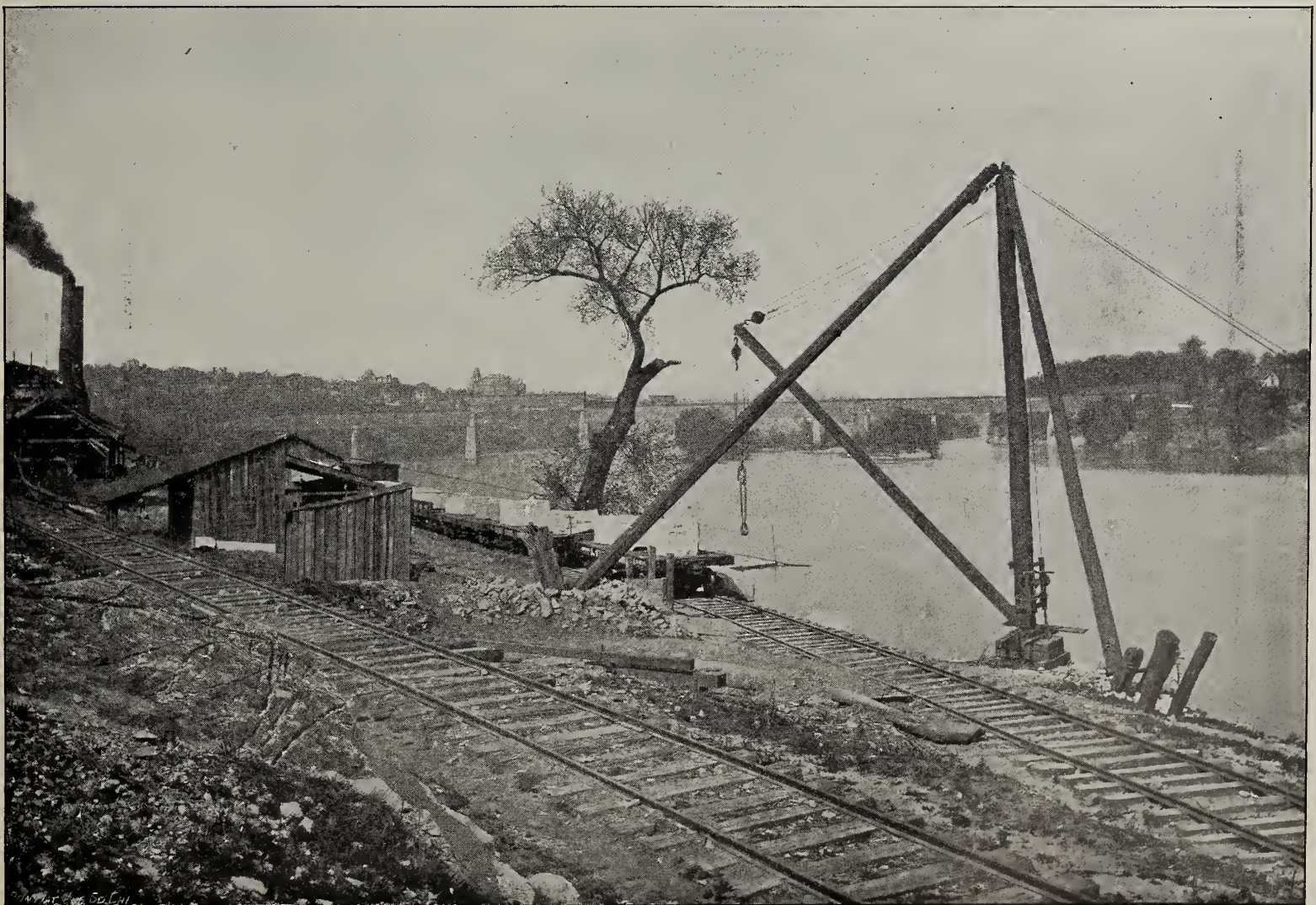
Derrick for Loading and Unloading Marble on the Tennessee, Knoxville.
