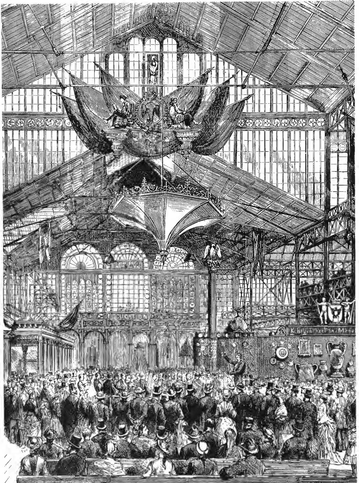
Music Pavilion, Central Transept, Main Building.
