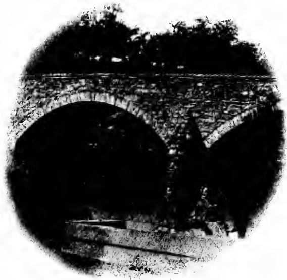
AT ANTIETAM BRIDGE
