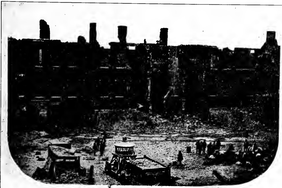
INTERIOR FACE OF GORGE. Showing Officer's Quarters and Gateway.
