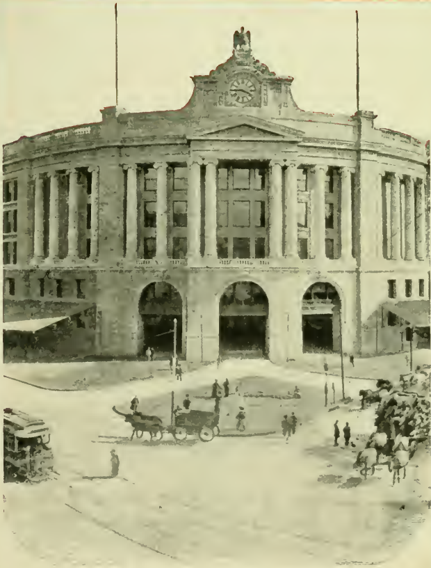
South Terminal Station
