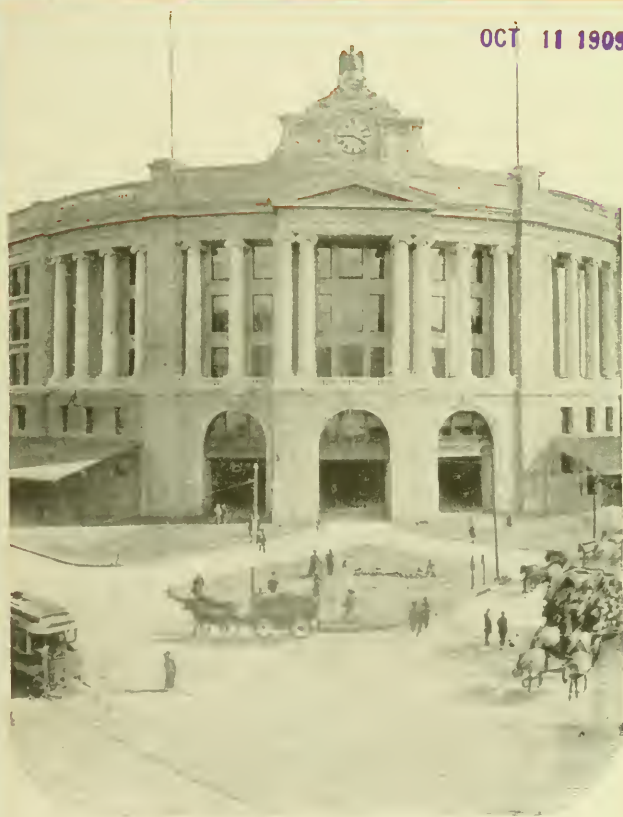
South Terminal Station
