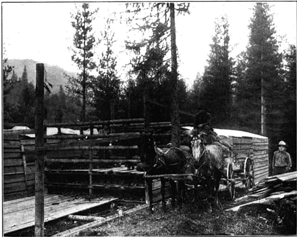
A PARTIALLY UNLOADED WAGON AT THE CONE BINS, SHOWING CONSTRUCTION OF BINS TO INSURE VENTILATION. [A boy tallied the sacks by the number of the pickers.]
