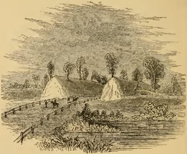
GRADED WAY IN OHIO.
