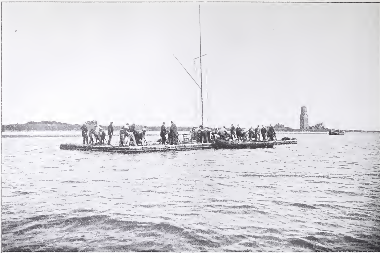
Fig. 30. Zinken in twintig meter water.
