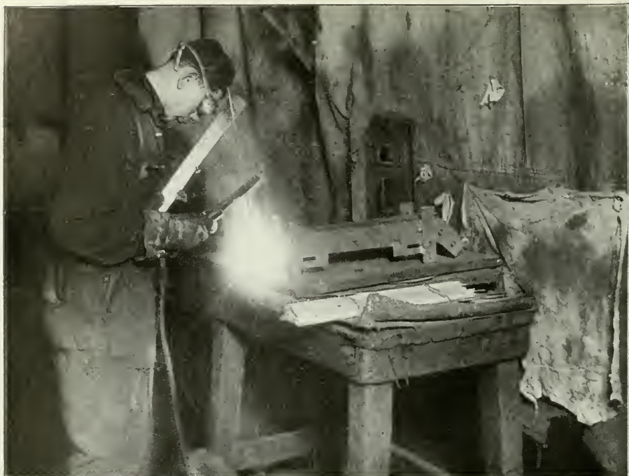
ACETYLENE WELDING ON PRESSED STEEL
