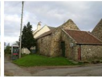
Stepped sides of buildings in Hart Village
