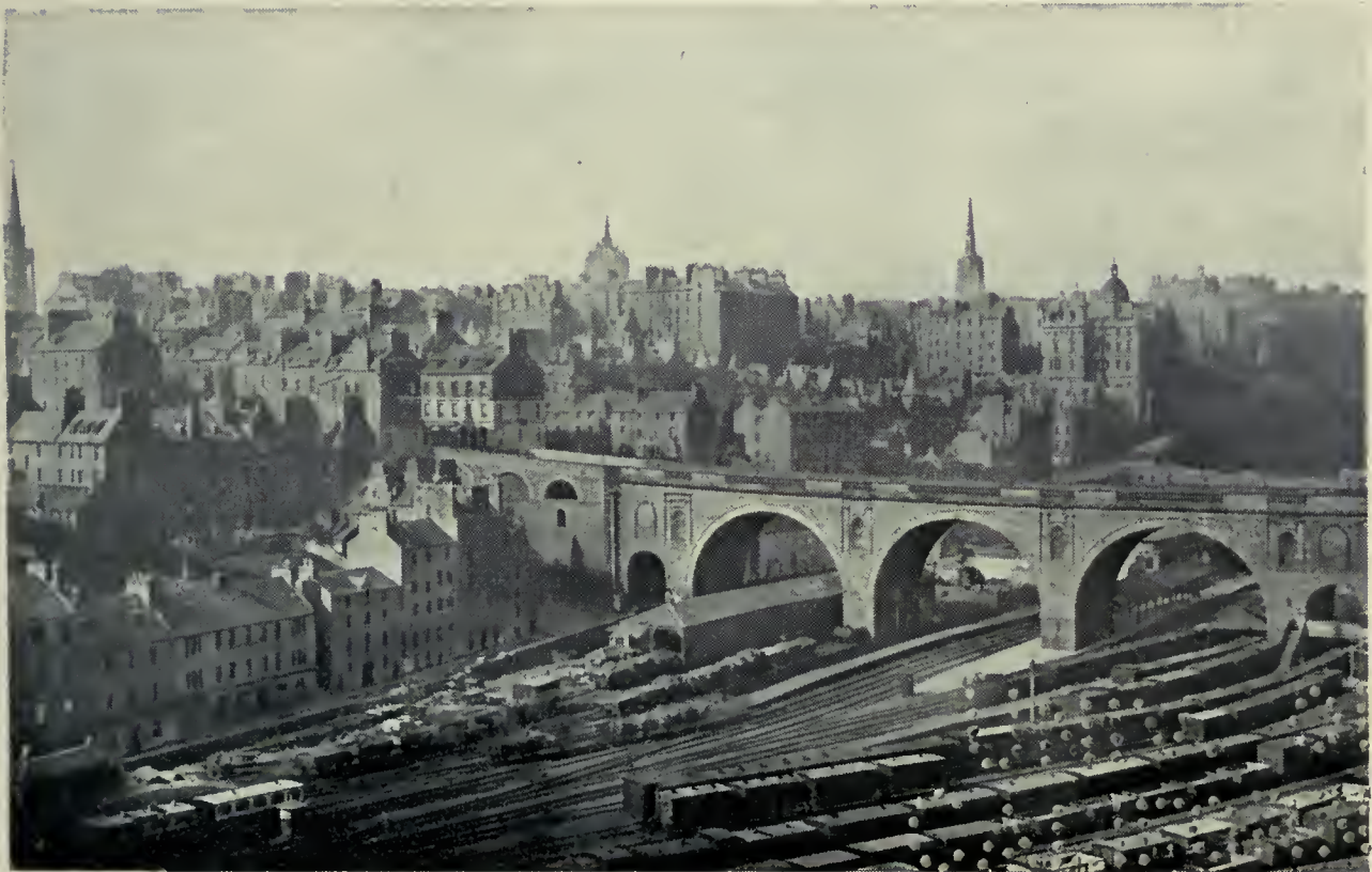
THE NORTH BRIDGE, WITH THE RAILWAY.
