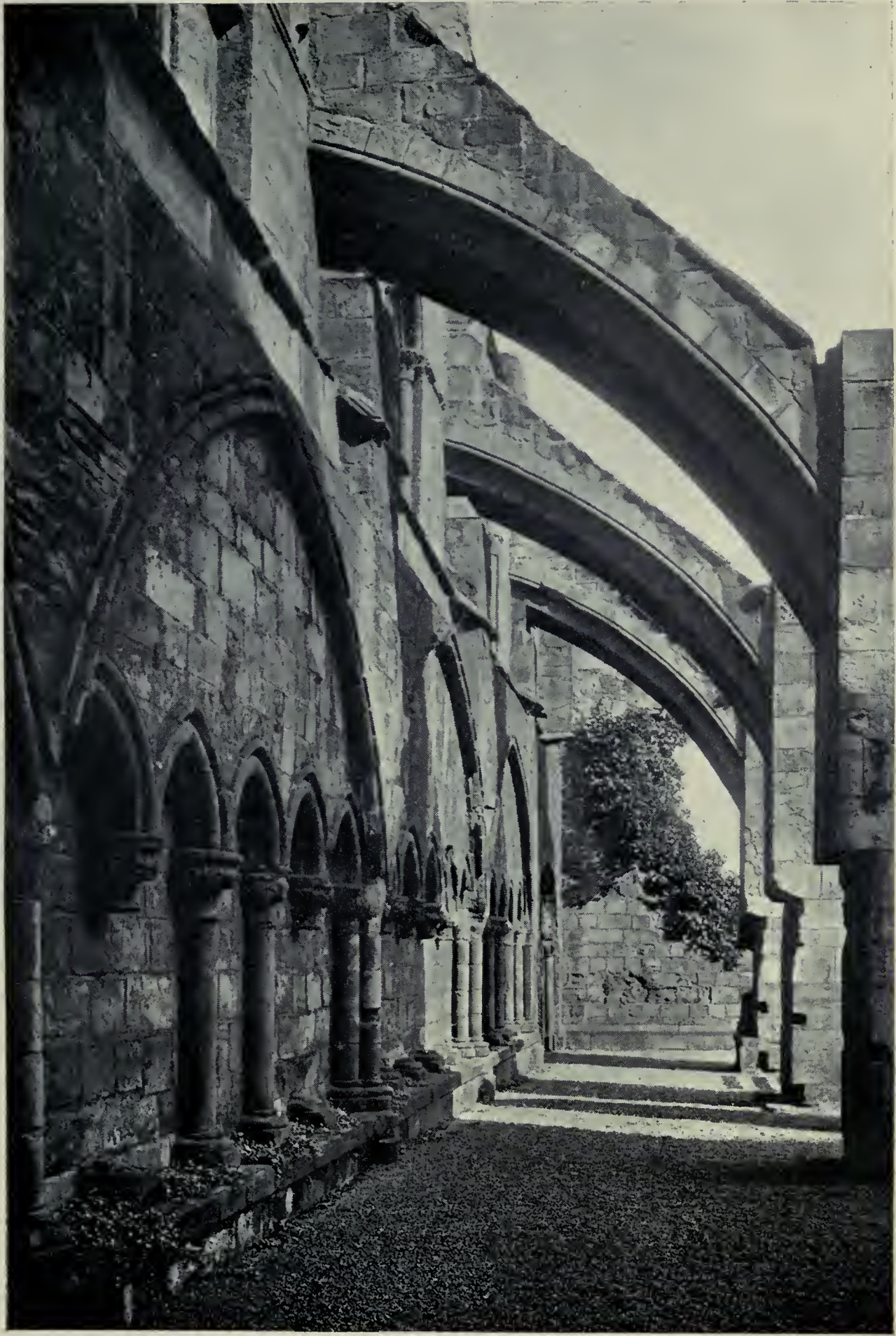
HOLYROOD ABBEY CHURCH REMAINS OF THE CLOISTERS.
