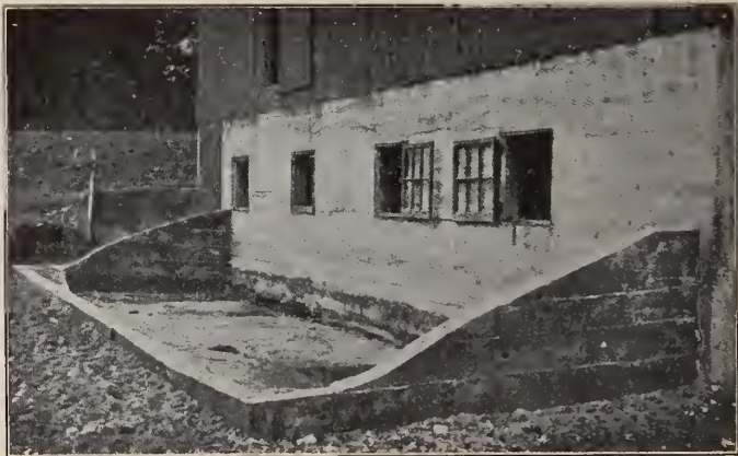
Concrete Manure Pit
