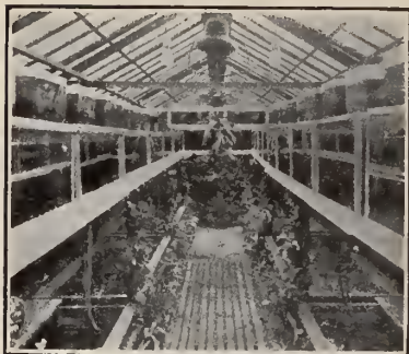
Low Span Greenhouse Used as a propagating pit. Note the glazed cases
