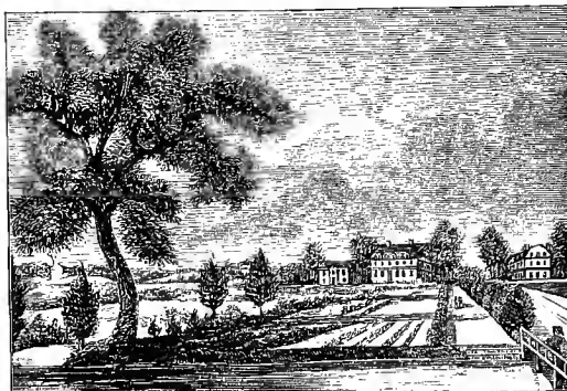
CLARKE'S HALL AND DOCK CREEK. [From an old drawing in Philadelphia Library.]
