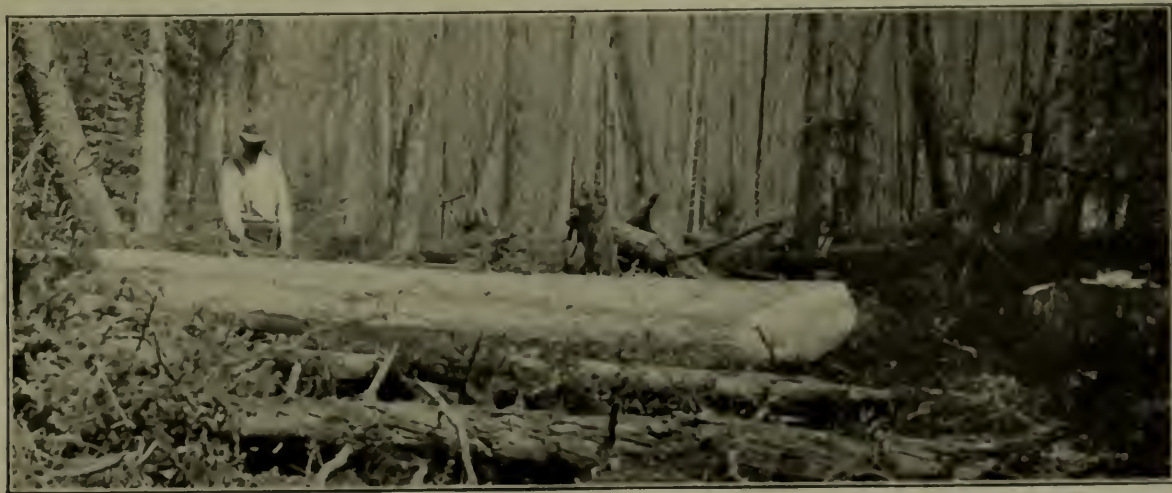
STARTING IN TO EXCAVATE THE HULL.
