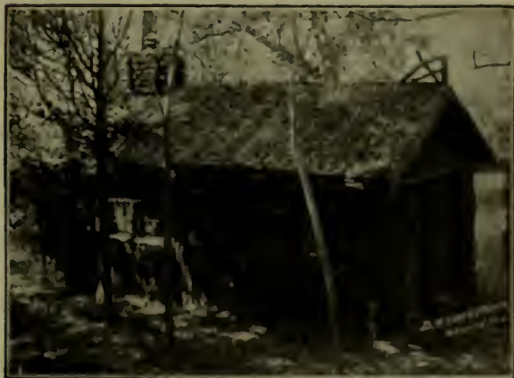
No. 3.—AUTOMOBILE HOUSE on Howard Gould's Estate, Sand Point, L. I. This house is suitable for either high or low site, as shown. Special designs furnished to suit your grounds free of charge. Built of best red cedar.
