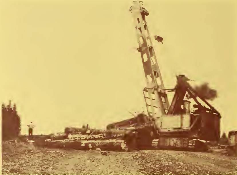
Figure 12.—Landing adjacent to road consisting of widened subgrade.
