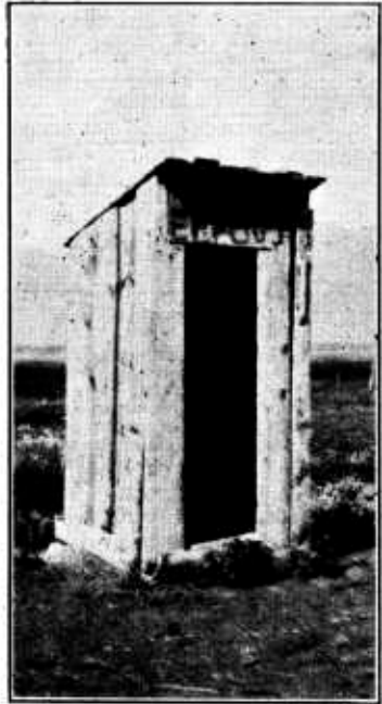
FIG. 2.—The rickety, uncomfortable, unspeakably foul, dangerous ground privy. Neglected by the owner, shunned by the hired man, avoided by the guest, who, in preference goes to near-by fields or woods, polluter of wells, meeting place of house flies and disease germs, privies of this character abide only because of man's indifference
