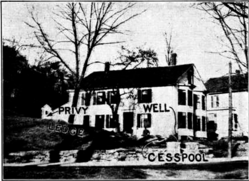
FIG. 5.—Poor relative locations of privy, cesspool, and well. (State Department of Health, Massachusetts.) Never allow privy, cesspool, or sink drainage to escape into the plot of ground from which the water supply comes
