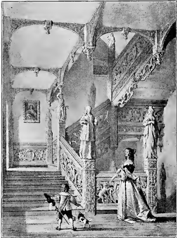
STAIRCASE, ALDERMASTON, BERKSHIRE.
