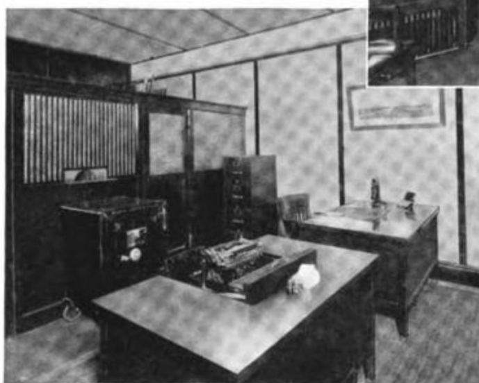
INTERIOR VIEW OF OFFICE
