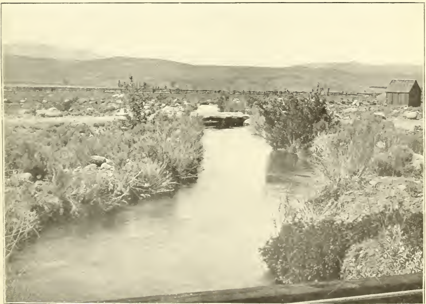
FIG. 2.—NEVADA STATION—IRRIGATION DITCH.
