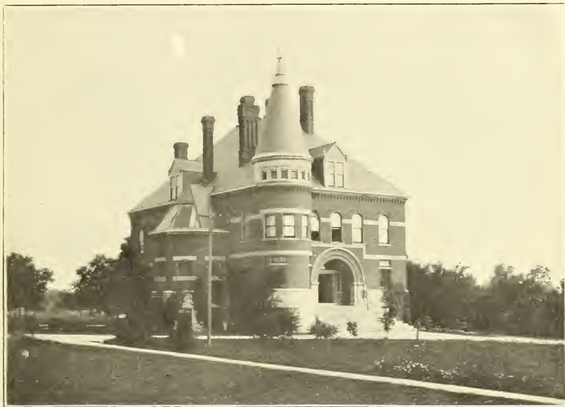
FIG. 1.—KENTUCKY STATION—MAIN BUILDING.
