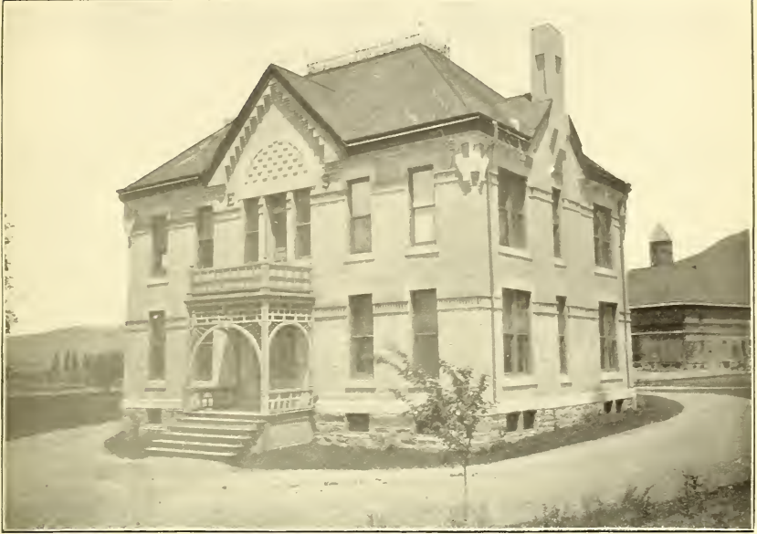
FIG. 1.—UTAH STATION—OFFICE BUILDING.
