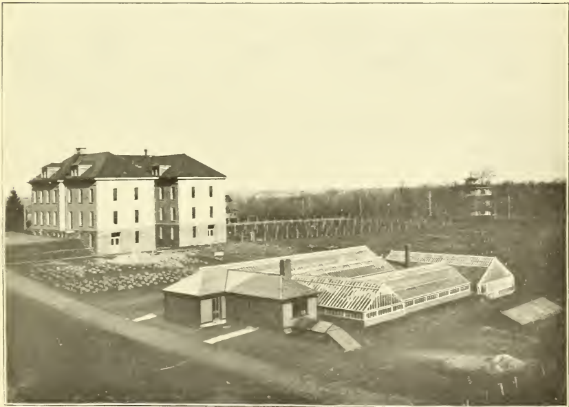
FIG. 2.—NEW YORK STATE STATION—FORCING HOUSES.
