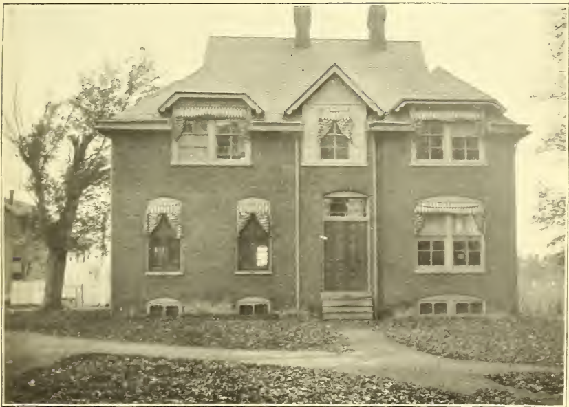
FIG. 2.—DELAWARE STATION—MAIN BUILDING.
