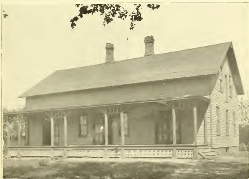
FIG. 2.—ILLINOIS STATION—HORTICULTURAL BUILDING.
