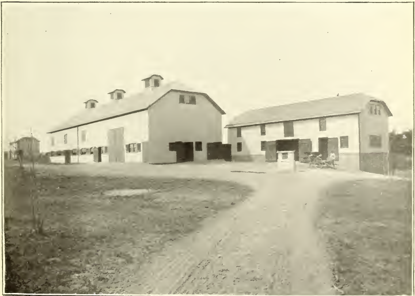
FIG. 2.—NEW JERSEY STATIONS—BARN.
