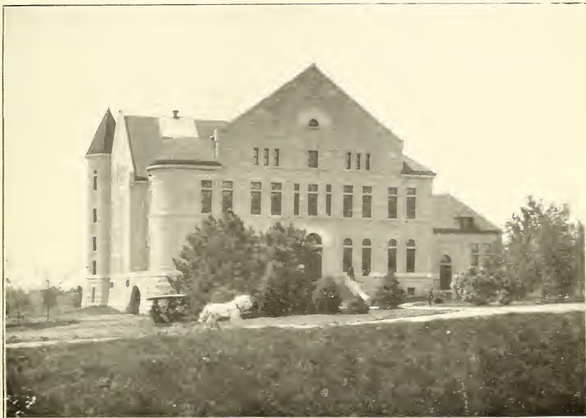
FIG. 1.—KANSAS STATION—LIBRARY AND AGRICULTURAL SCIENCE HALL, USED BY COLLEGE AND STATION.
