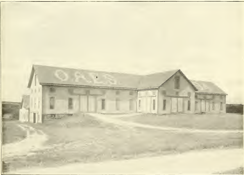
FIG. 2.—OHIO STATION—GRAIN AND DAIRY BARN.
