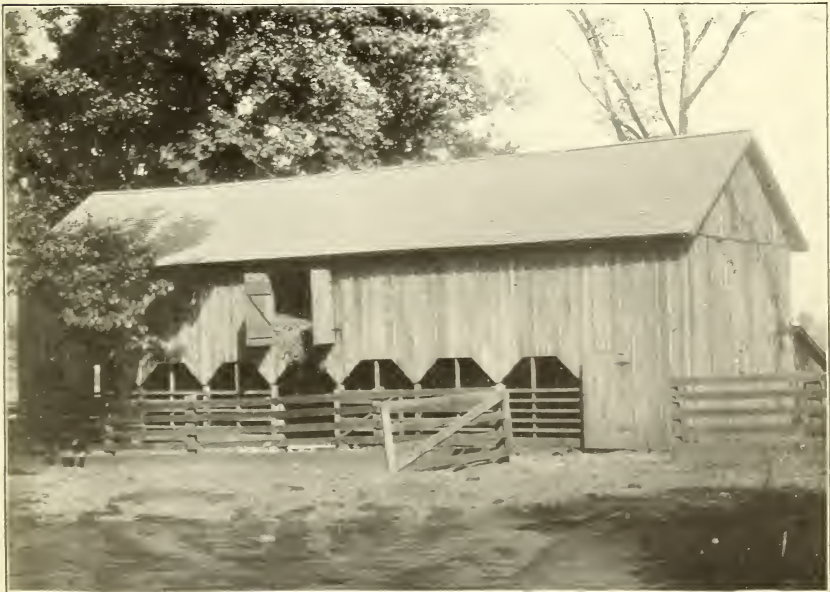
FIG. 2.—MISSISSIPPI STATION—CATTLE BARN.
