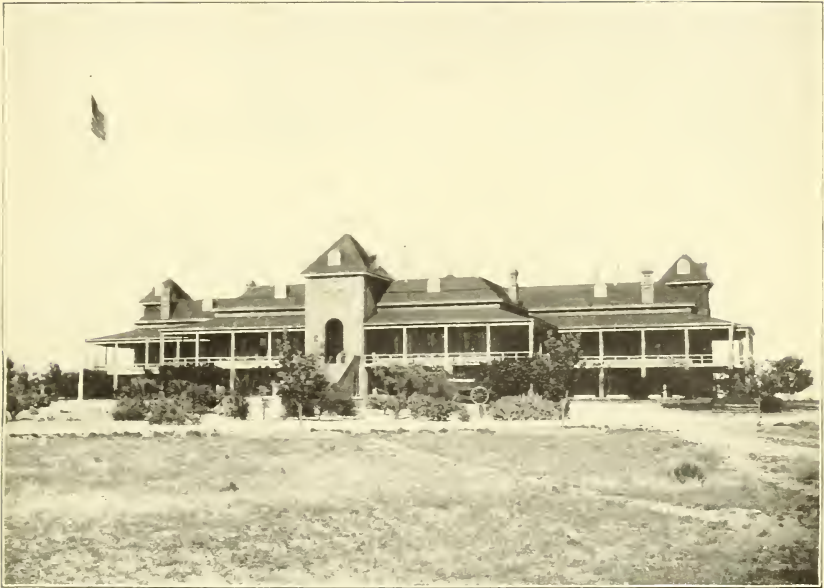
FIG. 1.—ARIZONA STATION—MAIN BUILDING, USED BY COLLEGE AND STATION.
