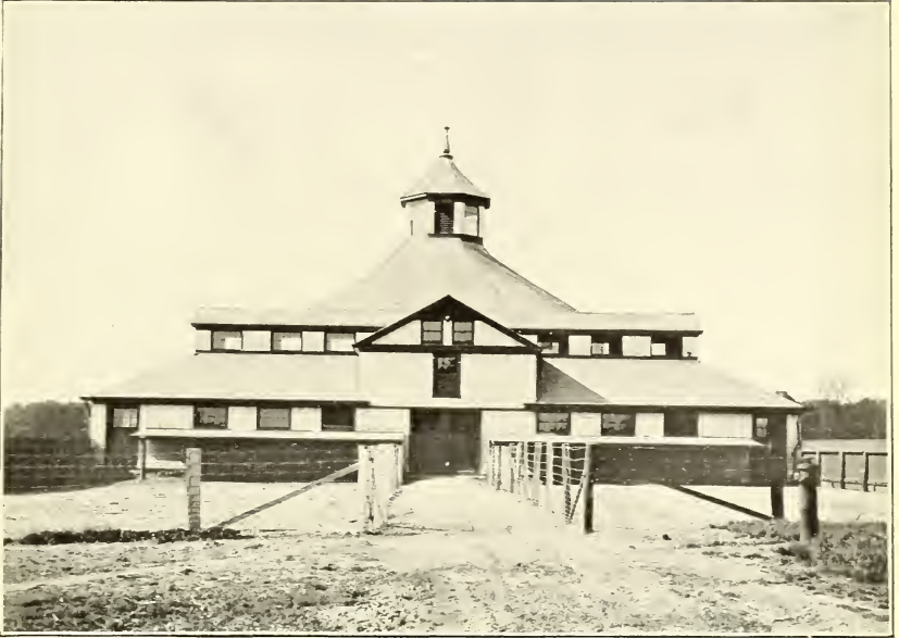
FIG. 1.—RHODE ISLAND STATION—BARN, USED BY COLLEGE AND STATION.
