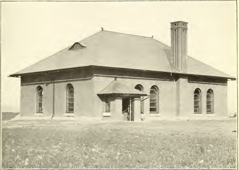
FIG. 1.—PENNSYLVANIA STATION—CALORIMETER BUILDING.
