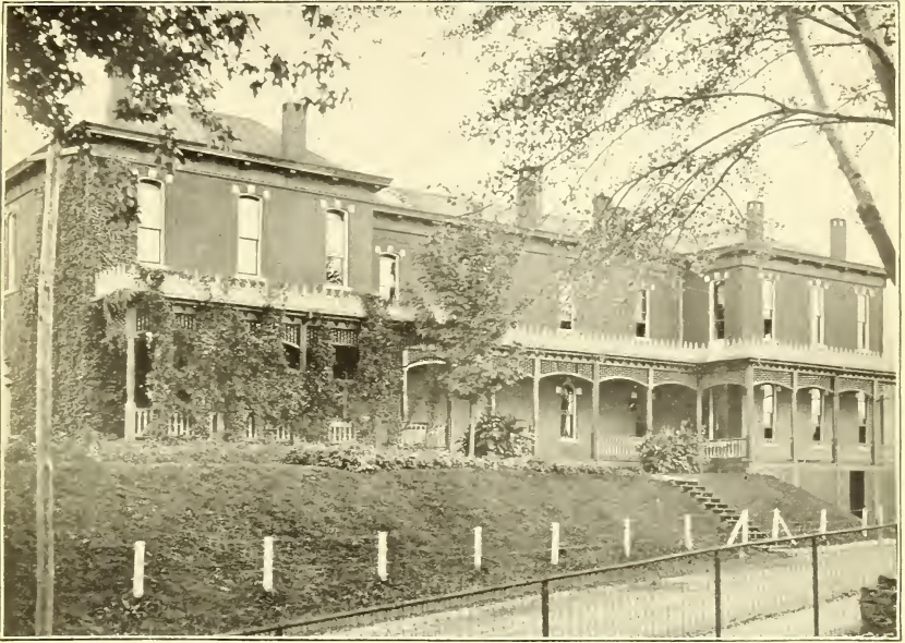
FIG. 1.—WEST VIRGINIA STATION—MAIN BUILDING.
