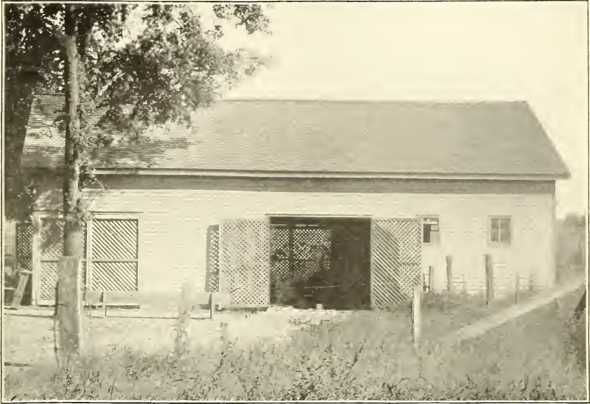
FIG. 1.—MISSISSIPPI STATION—TOOL BARN.
