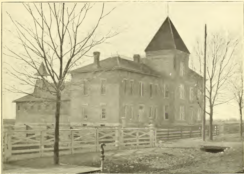
FIG. 1.—INDIANA STATION—AGRICULTURAL BUILDING.
