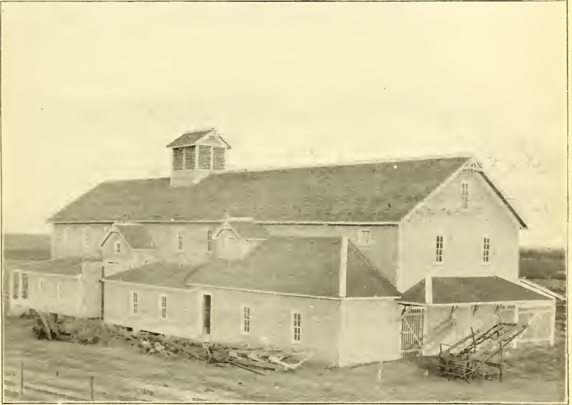
FIG. 2.—TEXAS STATION—MAIN BARN.
