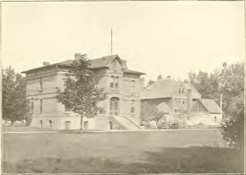
FIG. 1.—COLORADO STATION—IRRIGATION BUILDING, USED BY COLLEGE AND STATION.
