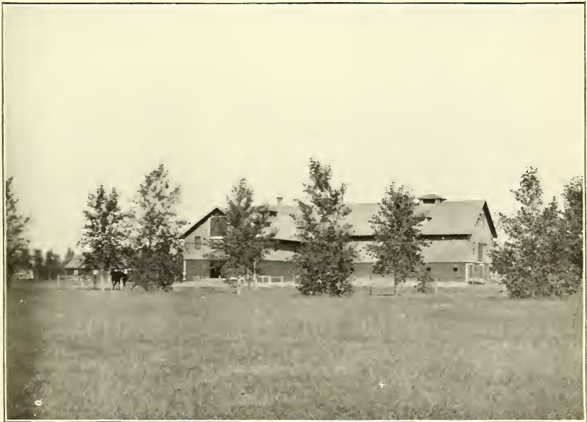
FIG. 2.—NORTH DAKOTA STATION—BARN.
