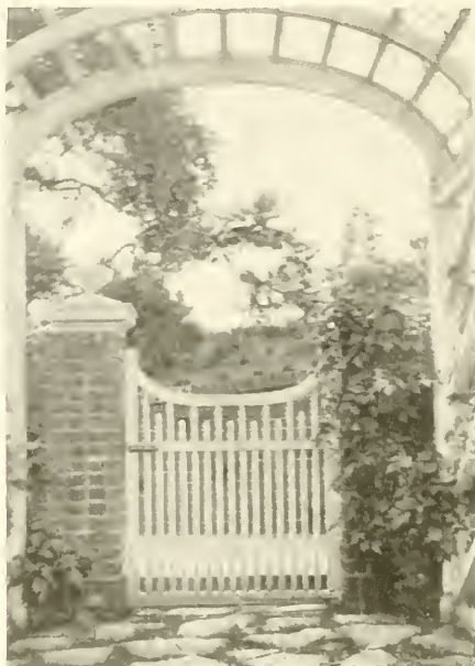
A GATEWAY AND ARBOR AT HAMILTON FARM
