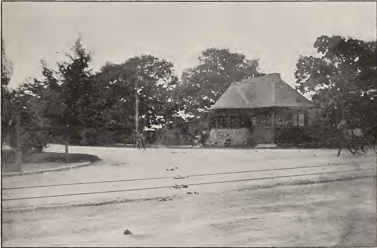
BROAD STREET ENTRANCE. On line of the Broad Street and Pawtuxet Trolley.
