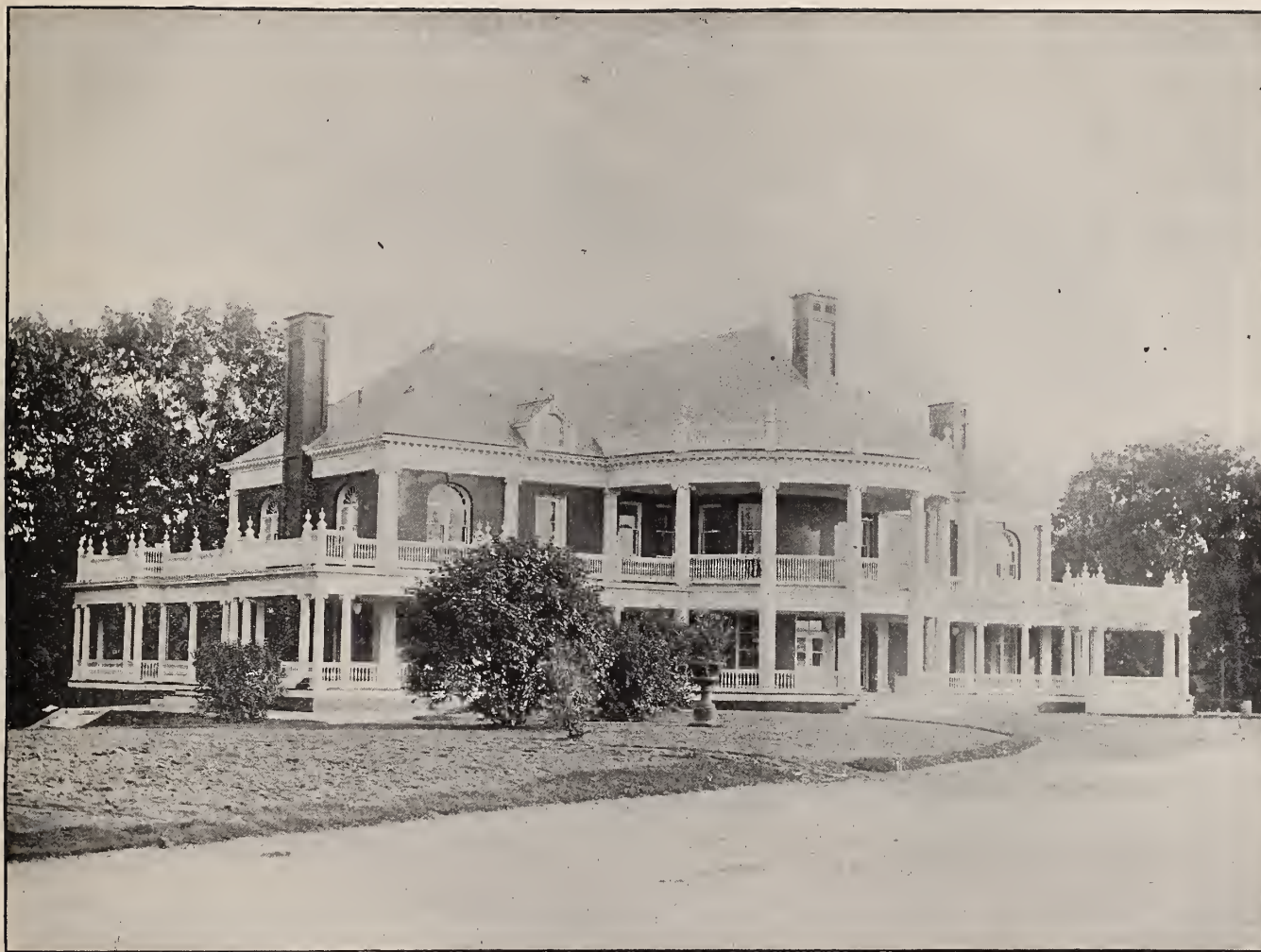
THE CASINO — NORTH FRONT.
