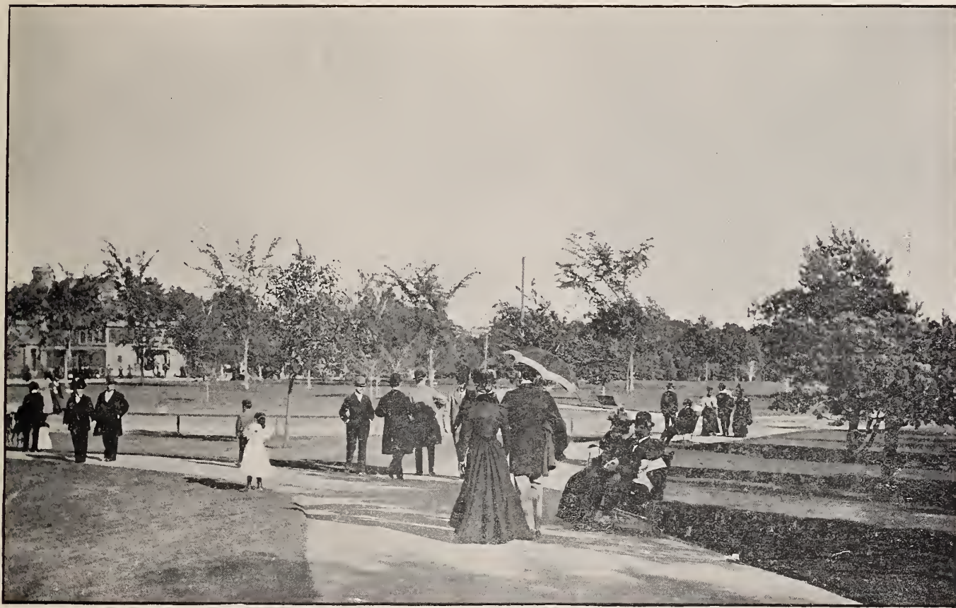
THE ELMWOOD AVENUE ENTRANCE.
