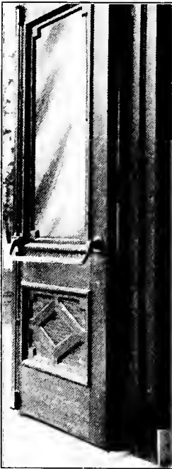
SCHOOL DOOR EQUIPPED WITH PANIC BOLT
