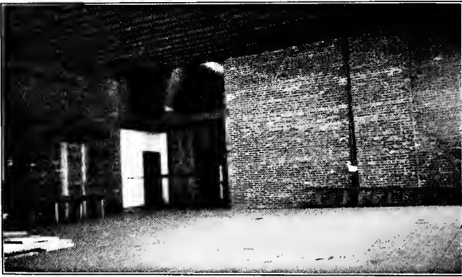
UNFINISHED AUDITORIUM IN THE BUNN SCHOOL ERECTED 12 YEARS AGO
