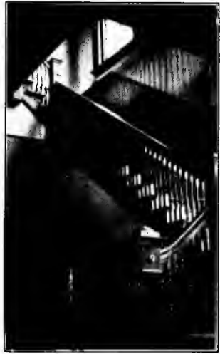
STAIRWAY OF DANGEROUS TYPE FOUND IN FEITSHANS SCHOOL
