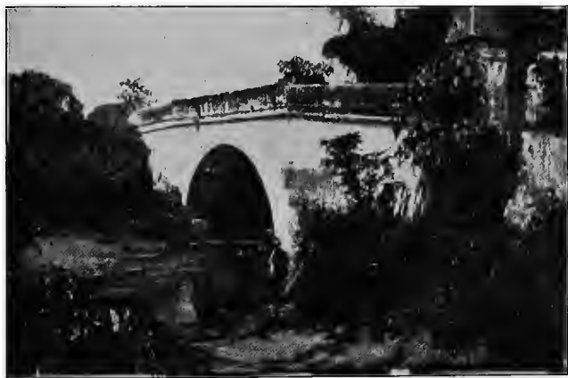
BRIDGE ON THE EL CANEY ROAD.
