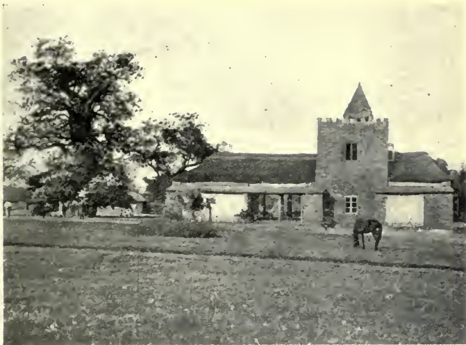
STATION AT BESSARI.
