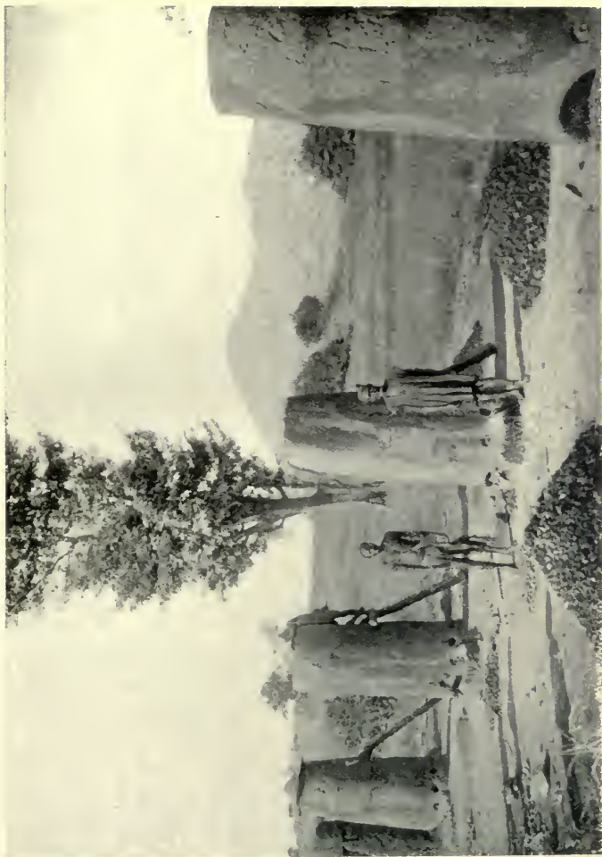
OVENS USED BY THE NATIVES FOR SMELTING IRON ORE AT BANGJELI, NORTH TOGO.
