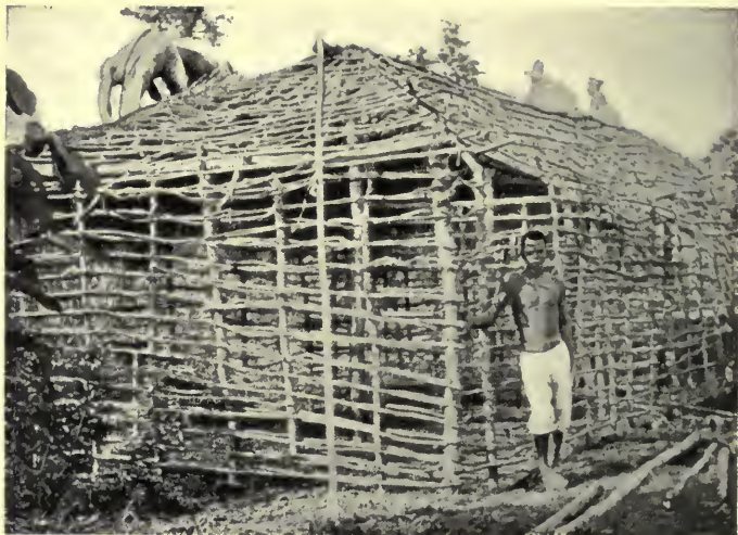
HOUSE, WITH GABLED ROOF, IN COURSE OF CONSTRUCTION. PLATE 119.
