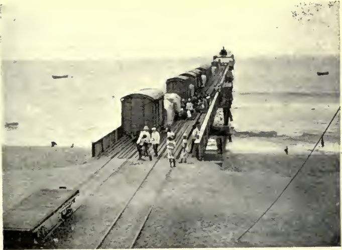
THE DESTROYED LANDING STAGE, LOME.
