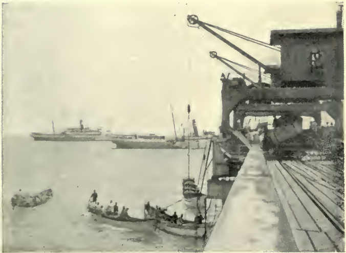
LANDING STORES ON THE BRIDGE, LOME.
