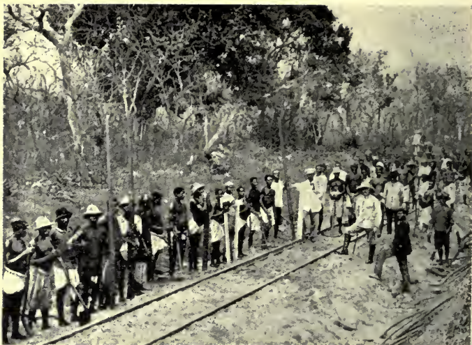
CONSTRUCTING THE RAILWAY TO ATAKPAME.
