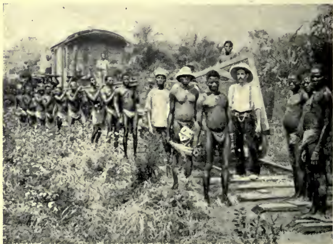
CONSTRUCTION OF THE HINTERLAND RAILWAY TO ATAKPAME.
