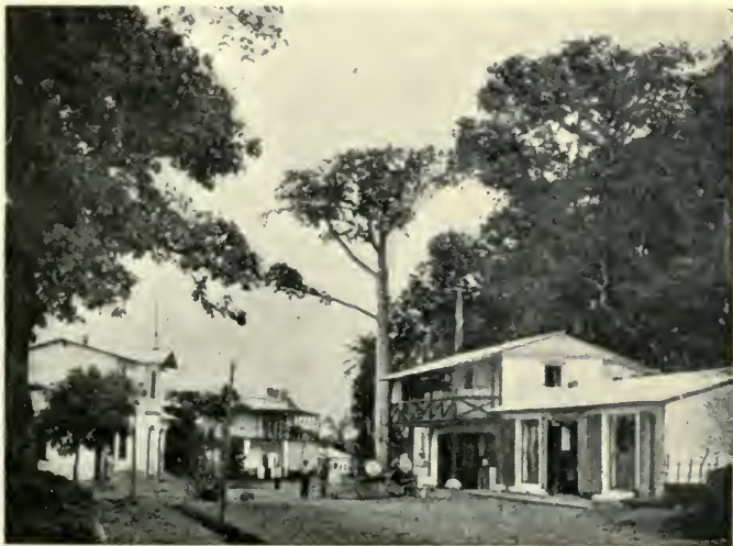
MISA HEIGHT STREET, PALIME.
