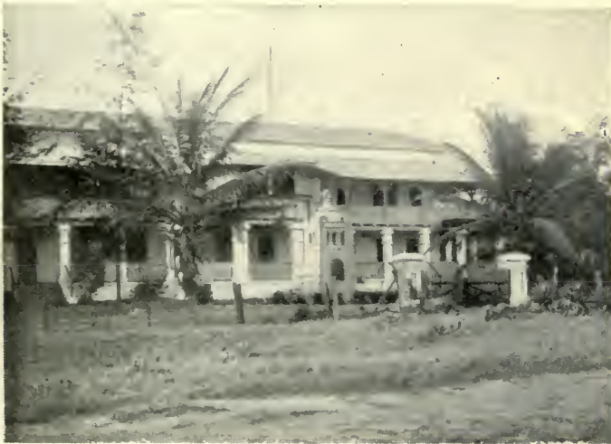
THE NIGHTINGALE HOSPITAL, ANECHO.
