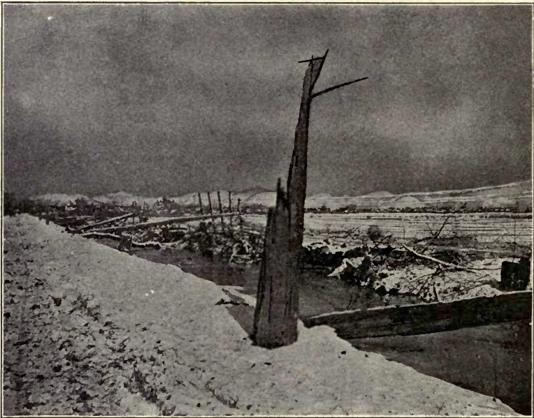
FIG. 139. — Effect of Sleet on Pole Line.
