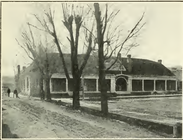
EXECUTIVE BUILDING, FORT STANTON, N.M.
