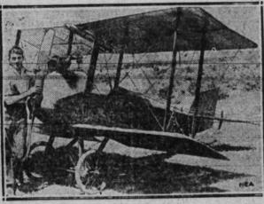
"BABY" PLANE RACE ENTRY—A baby aeroplane, which weighs but 228 pounds, has been entered in the race for light planes to be held during the International Air Races at Dayton, O. It has a wing spread of twelve feet and is propelled by a sixty-one cubic inch displacement motorcycle engine. Bert Mix, an aeroplane me-chanic of Dayton, built the machine, which can make about seventy-five miles an hour.
