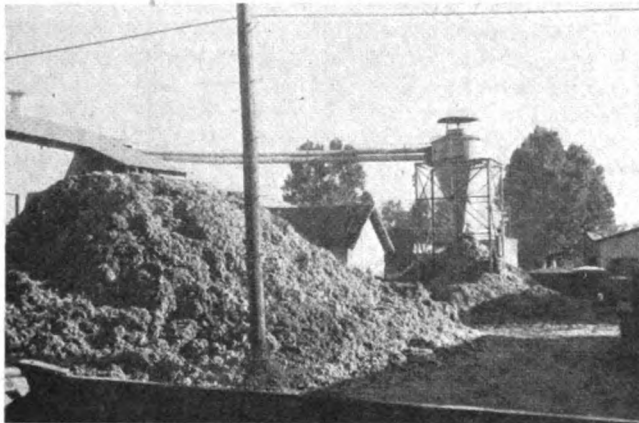
Trash and dust from cotton gins. —Cyclone dust collectors are used to settle dust from the discharged air, but some is still blown away. Gin workers may have transient effects from dust, but short seasonal operation prevents the more
