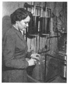
A sample of breath submitted by a manufacturer of radium-painted dials is being drawn off from a sampling flash in the radon testing laboratory at the National Bureau of Standards. After introduction into the ionization chamber (lower right), the radon content of the sample is measured by a count of the alpha particles which are emitted in the process of the disintegration of radon.
