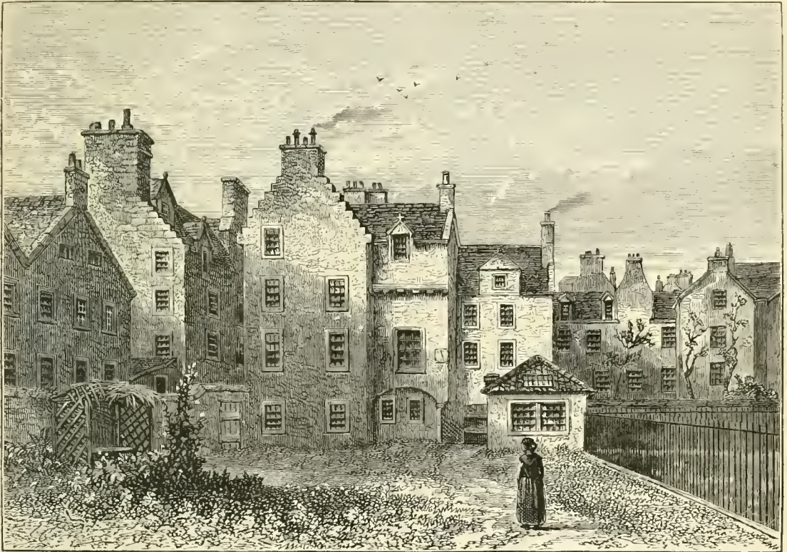
THE EARL OF SELKIRK'S HOUSE, WYNDFORD'S CLOSE (South view).
