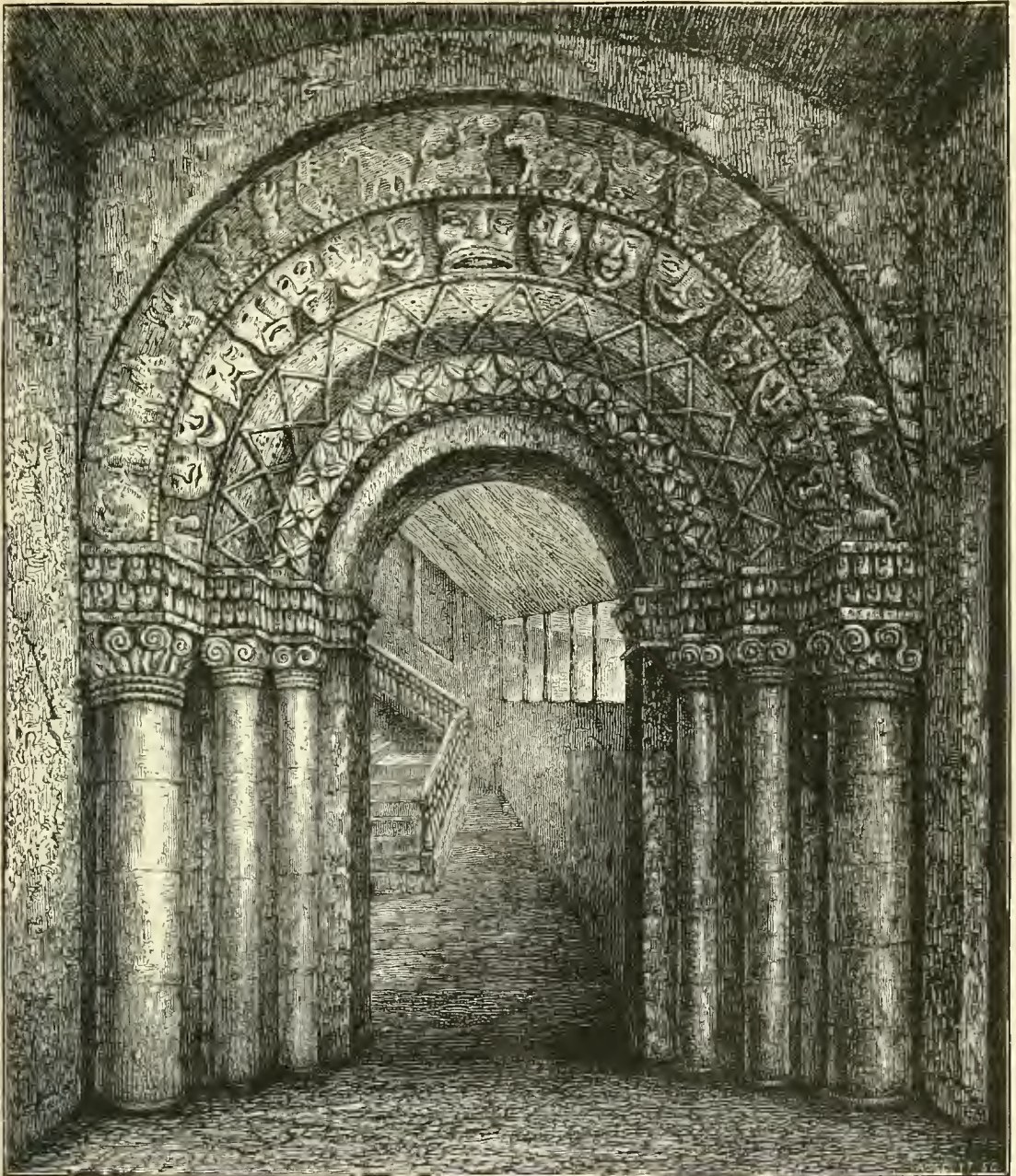
THE NORMAN DOORWAY, ST. GILES'S, WHICH WAS DESTROYED TOWARDS THE END OF THE EIGHTEENTH CENTURY. (From a Drawing by Armour about 1799.)
