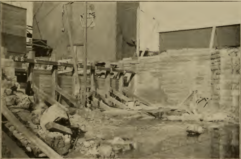
HEAD GATES—ROCKFORD GENERAL ELECTRIC CO.
