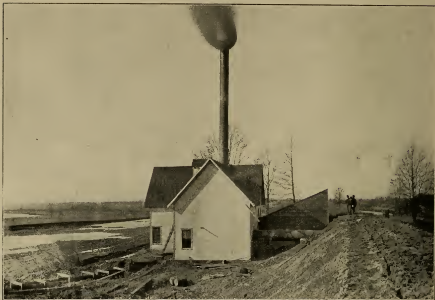
POWER STATION MEREDOCIA DRAINAGE DISTRICT.
