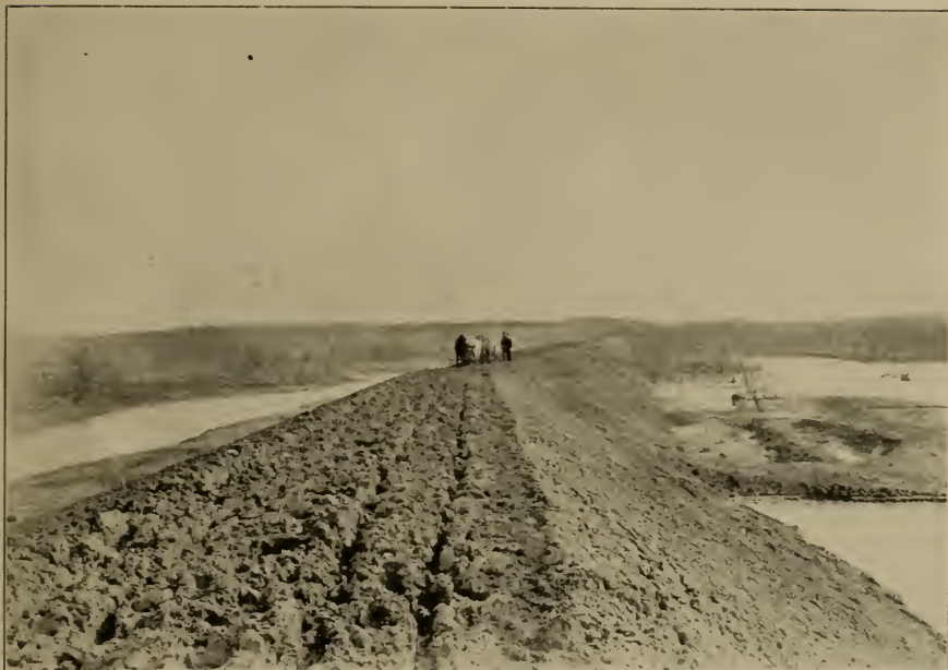
THE LEVEE—MEREDOCIA DRAINAGE DISTRICT.
