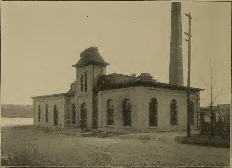
PUMP HOUSE—ROCKFORD, ILLINOIS.
