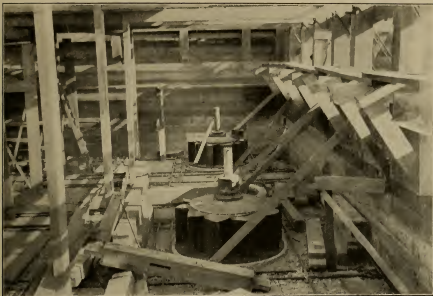
TWO WHEELS IN PLACE—ROCKFORD GENERAL ELECTRIC CO.
