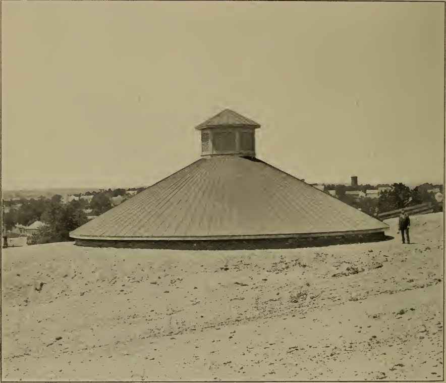
STORAGE RESERVOIR—WEST DUNDEE, ILL.
