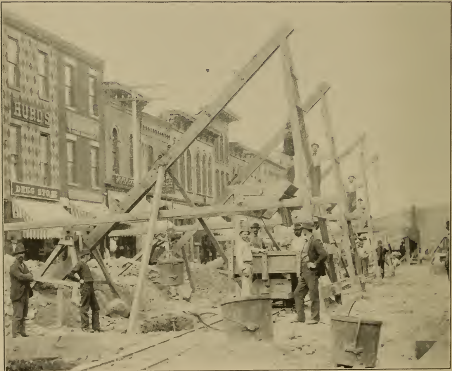
SEWER MACHINE AT WORK—AURORA, ILLINOIS.
